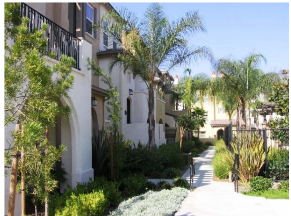
Multi-family housing units in 4S Ranch
