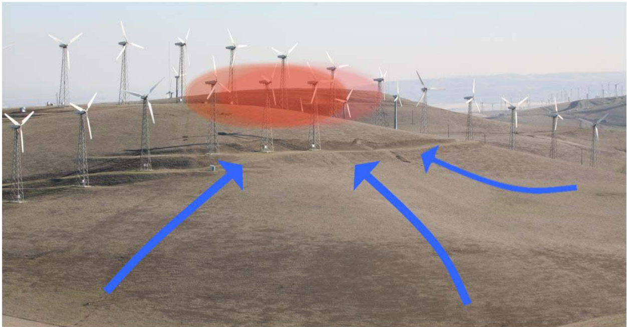
Photo 21. Wind turbines should not be relocated to locations on the slope where downslope hill morphology pushes the wind toward these locations from two different prevailing wind directions. In this photo, the red highlight identifies a portion of the air space where winds will be pushed to greater speeds by winds blowing from the northwest, west, southwest, and south.
