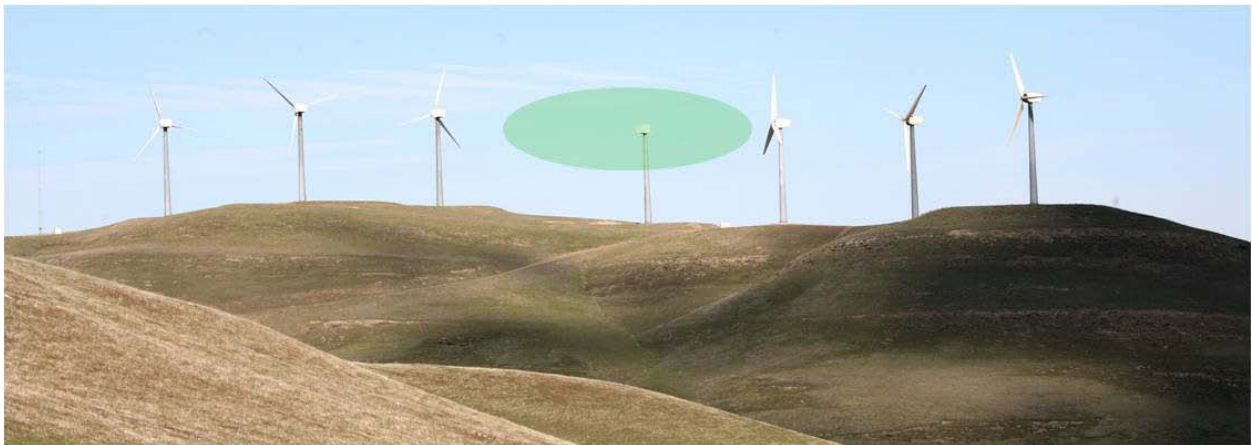
Photo 2. A derelict tower interior to the turbine row and at the top of the hill would be a relatively safer relocation site.
