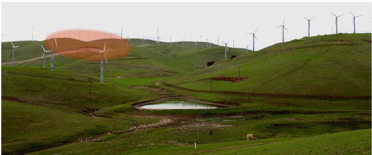
Photo 13. Wind turbines should not be relocated to saddles or to the lower aspects of a ravine or canyon, especially not next to a pond or stream.
