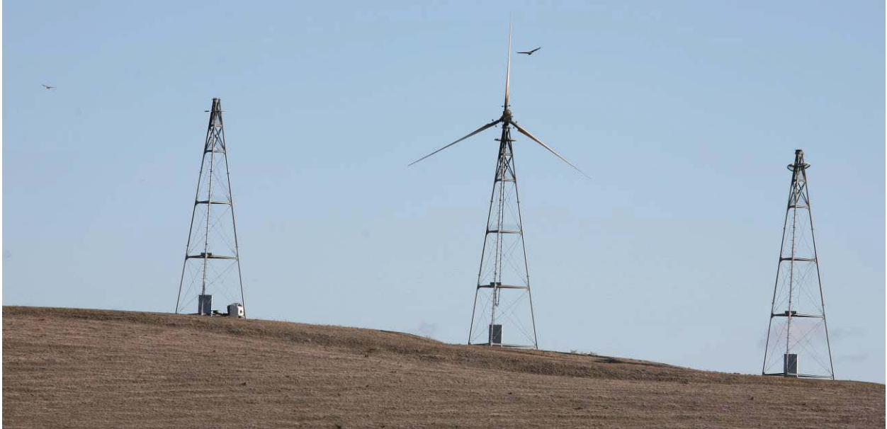
Photo 1. The two derelict towers to either side of this functional turbine on the ridge crest should either be removed or put back into service. If the derelict towers are removed, then the interior functional turbine should also be removed.
