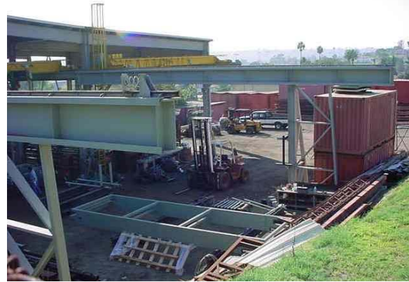
Steel fabricating plant in Spring Valley
