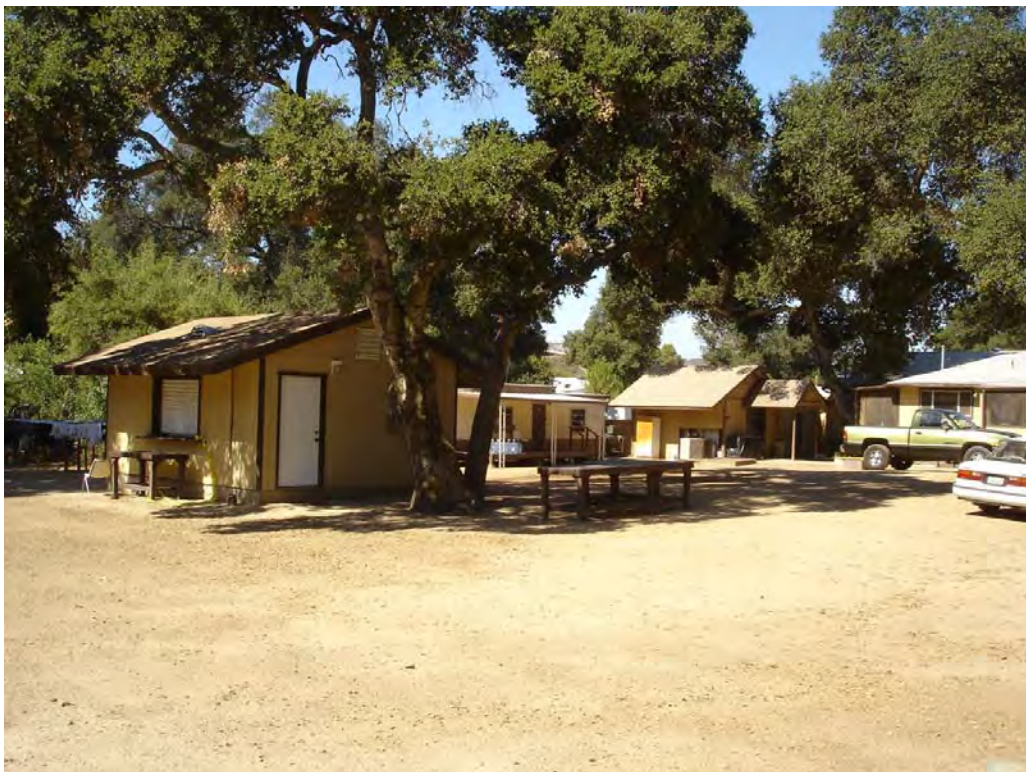
Photograph 2. View of existing structures in the central portion of the site
