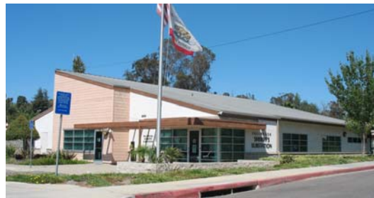
Fallbrook Sheriff substation
