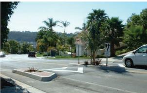
**Speed Hump or Speed Lump:** Similar to a speed bump, but wider and gentler. Speed “lumps” are speed humps with precisely spaced breaks allowing large (emergency) vehicles to pass without damage or slowing.
