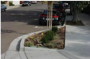
**Curb Extensions (“bulb-outs”):** Narrow the intersection or mid-block crossing distance by extending the curb into the street, making pedestrians more visible and reducing the speed of turning vehicles.
