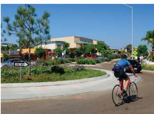
**Modern Roundabout:** A circular intersection median that more safely processes conflicting traffic without the need for stopping, while increasing street capacity using existing lanes.
