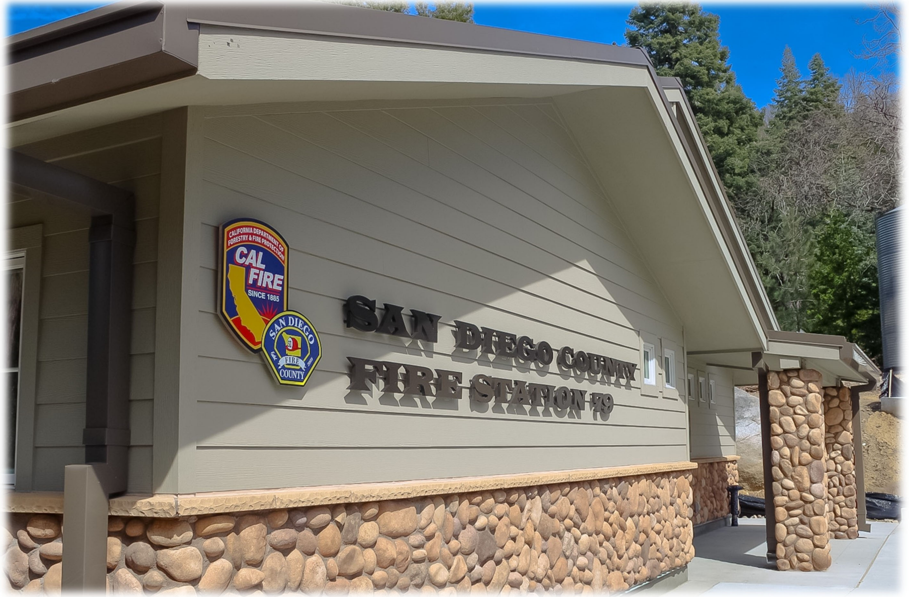
County Fire Station 79 includes newly added living quarters for firefighters serving Palomar Mountain.
