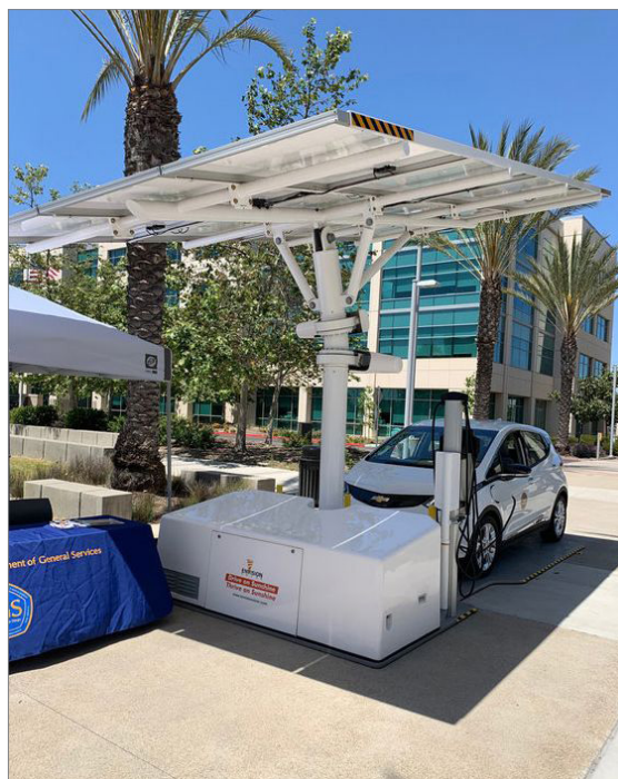
Photovoltaic charging unit at the County Operations campus for electric vehicles.
