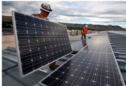
Worker installing rooftop solar panels
