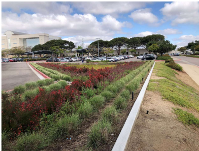
Drainage swale at the North County Regional Center in Vista
