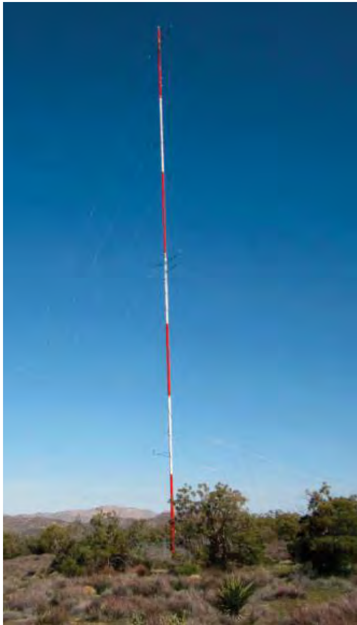
Photo 5: MET Towers are scattered across the landscape within the vicinity of the project area consisting of tubular towers that are approximately 200 feet in height.
