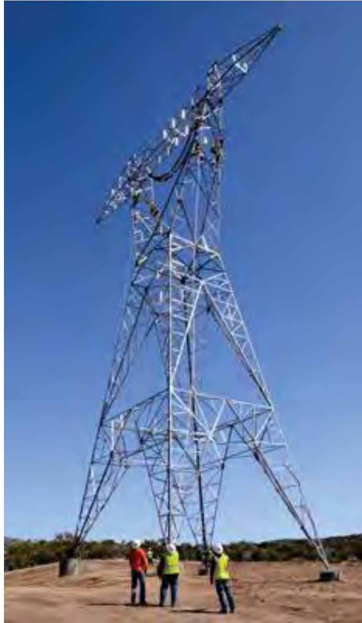
Photo 1: Sunrise Powerlink 500 kV Steel Lattice Towers are located immediately adjacent to the project site along McCain Valley Road.
