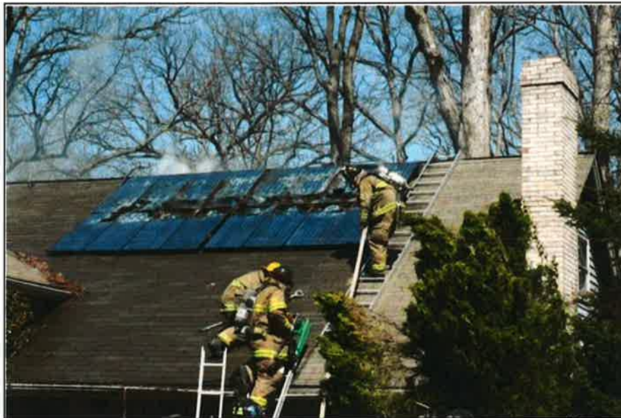
Figure 2-13: Residential PV Fire in March 2010 MD Incident 48
