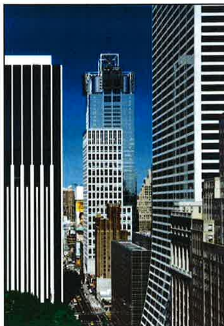
Figure 3-7: BIPV System Using a Vertical Module Configuration in New York City (Photo courtesy of NREL Photographic Information Exchange)
