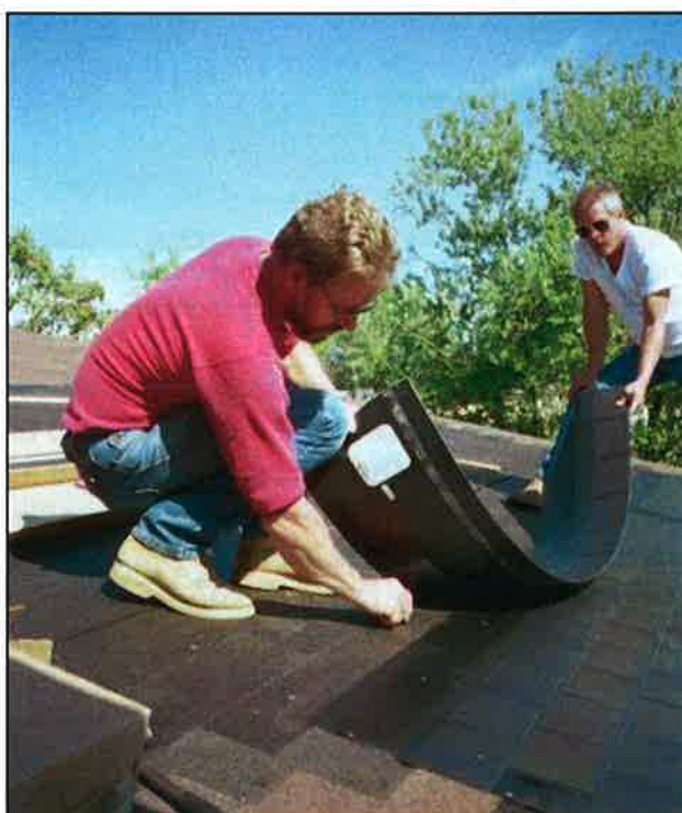
Figure 5-7: An Example of PV System Integral with Building Components (Photo courtesy of NREL Photographic Information Exchange)
