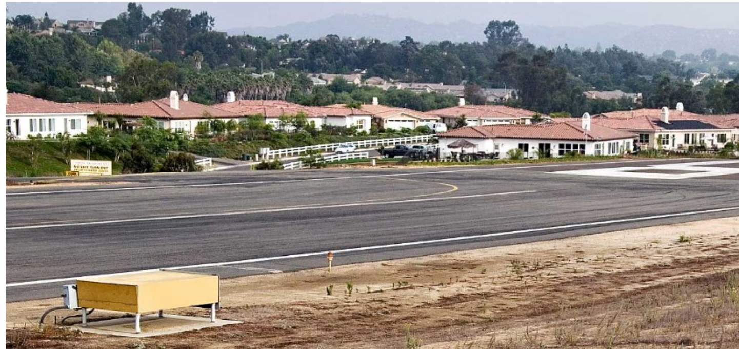
Figure 5 Fallbrook Airpark site photo
