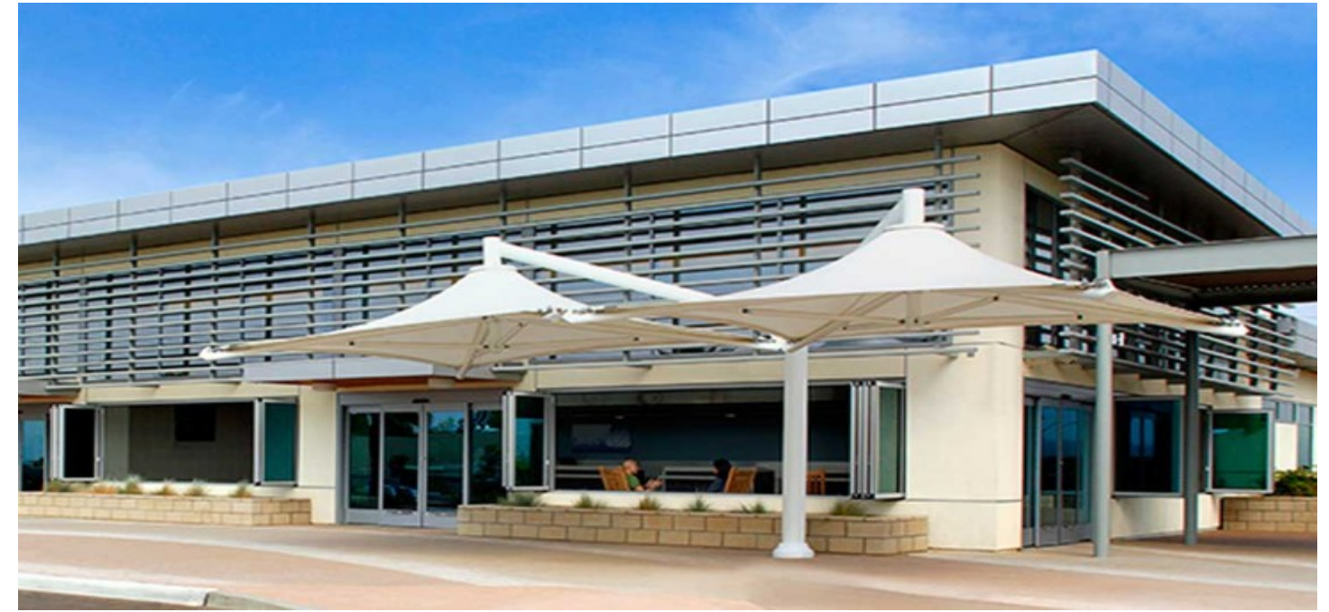
Figure 8 McClellan-Palomar Airport terminal building, built to LEED standards
