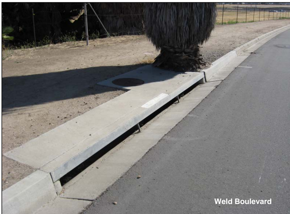
Photo A-1: Catch basin on Weld Boulevard that conveys off-site flows to Drainage A.
