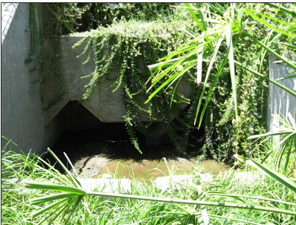
Photo F-1: Square concrete culvert and spillway that conveys off-site flows to Drainage F.
