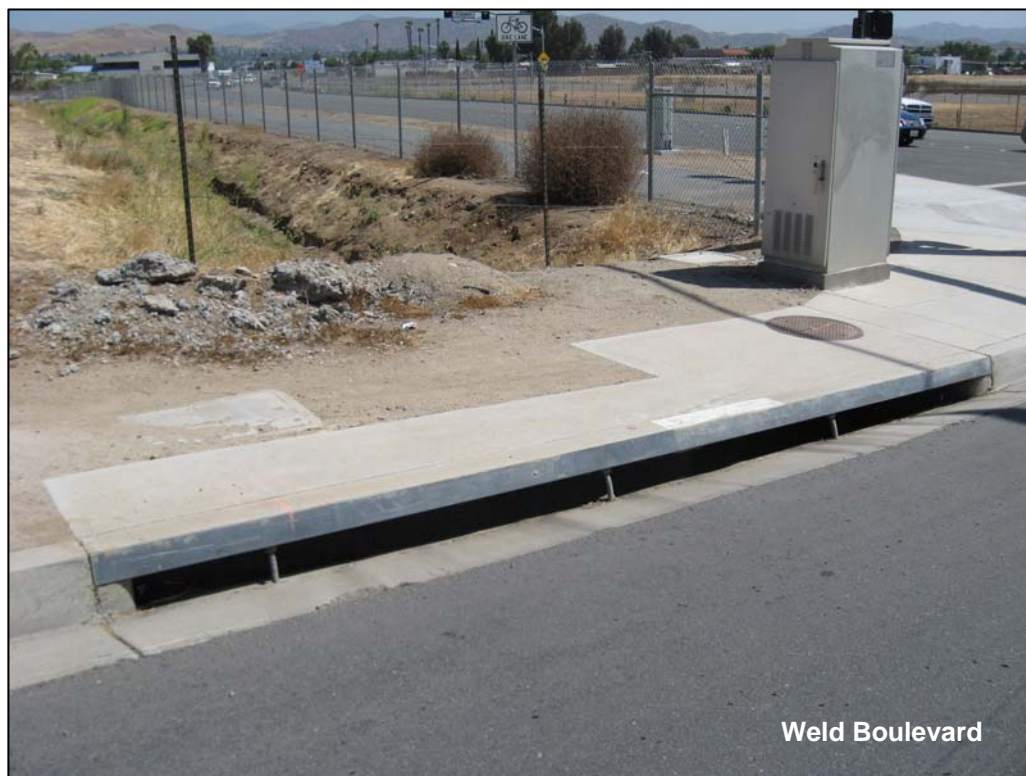
Photo B-1: Catch basin on Weld Boulevard that conveys off-site flows to Drainage B.
