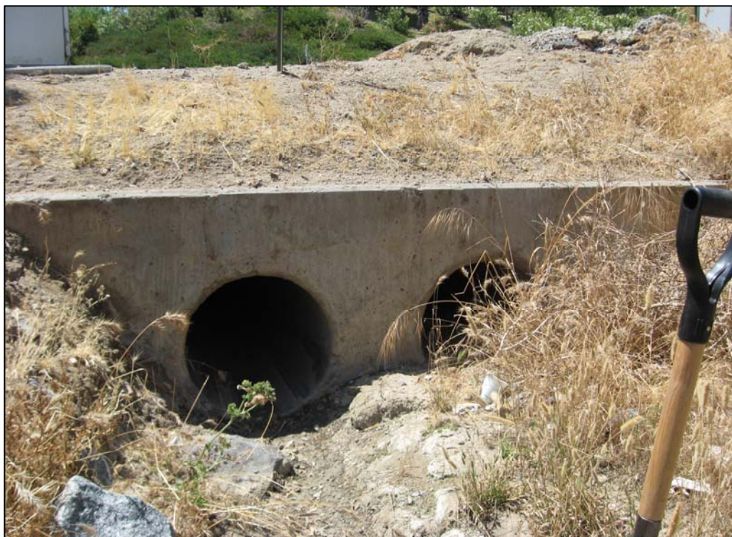
Photo B-2: Double concrete pipe culvert that conveys off-site flows to Drainage B, looking south. The bottom one-third of the western pipe (on right) is filled with sediment. Channel is centered on the eastern pipe (on left).
