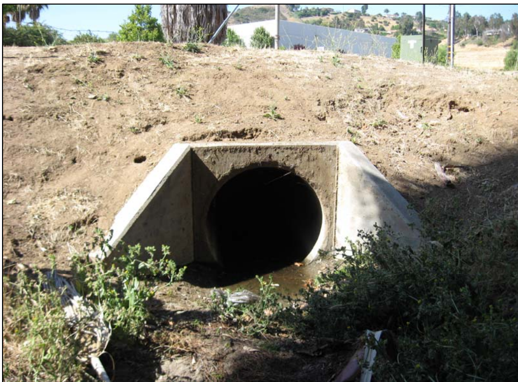
Photo A-2: Thirty-six inch concrete pipe culvert that conveys off-site flows to Drainage A.
