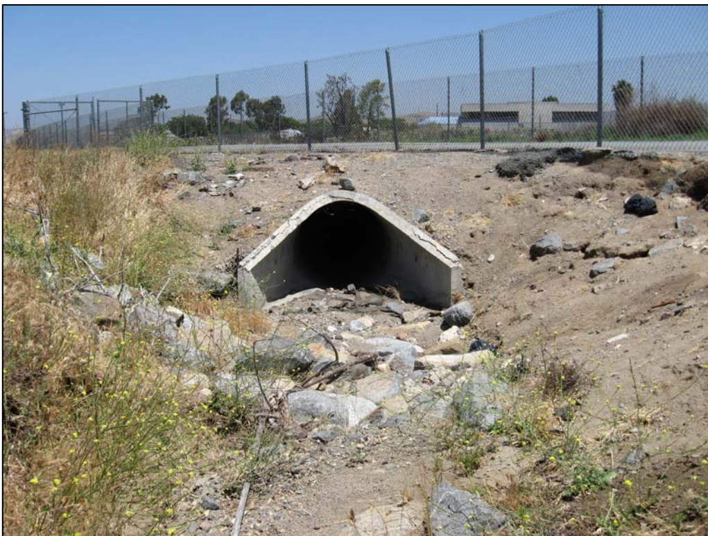
Photo C-4: Thirty-six inch concrete culvert located at the terminus of Drainage C. This culvert conveys flows from Drainage C to Forrester Creek.
