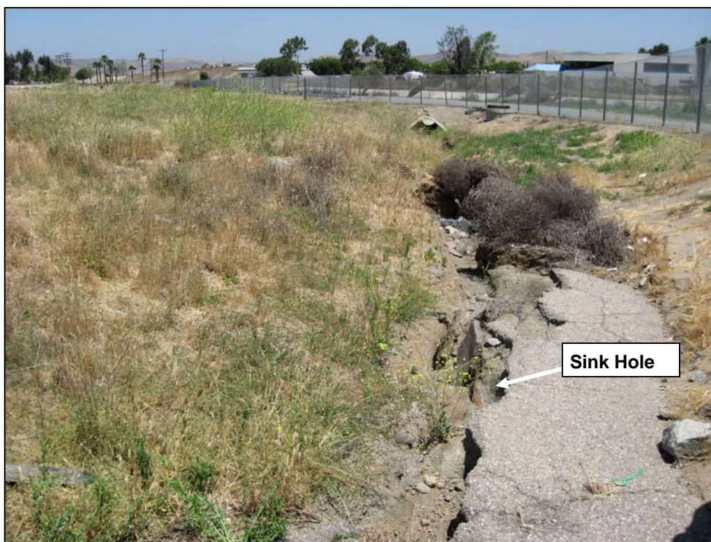
Photo C-2: Fifteen foot long by one foot wide asphalt sinkhole at terminus of Drainage C. Culvert at terminus of Drainage C can be seen in the background.
