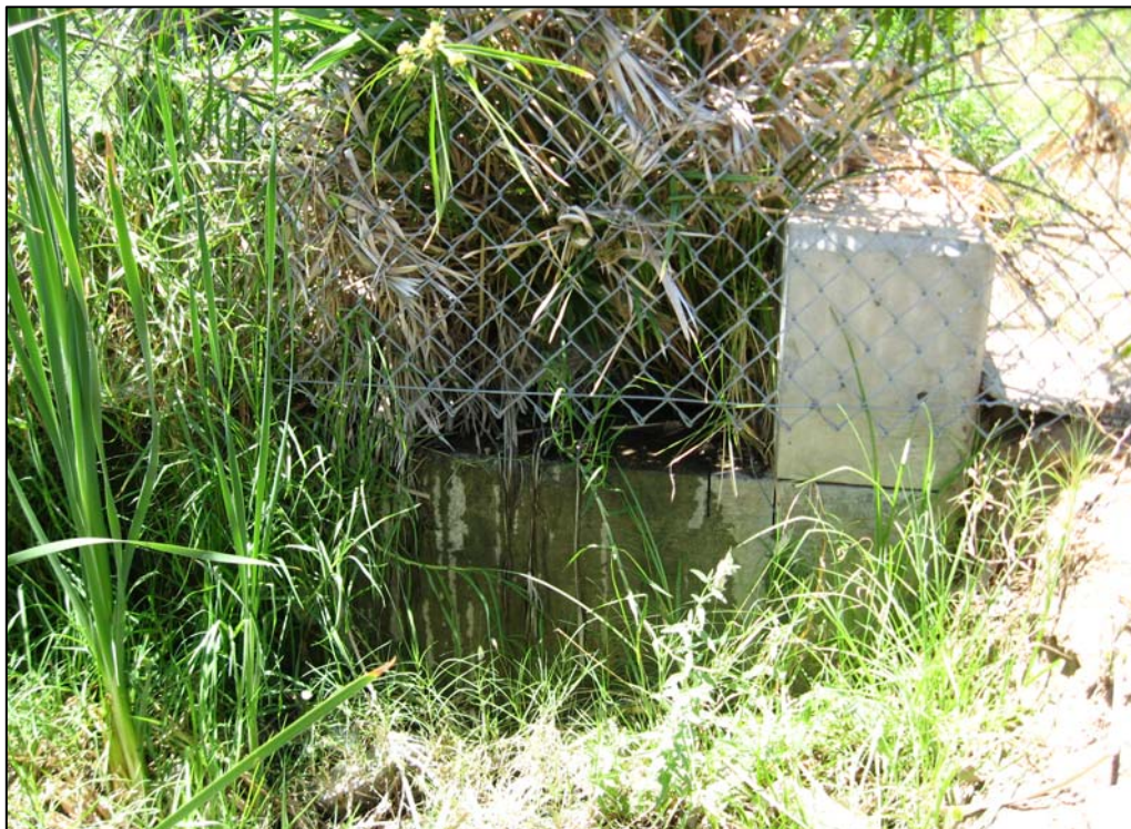
Photo F-2: Water is present in Drainage F due to overtopping of spillway.
