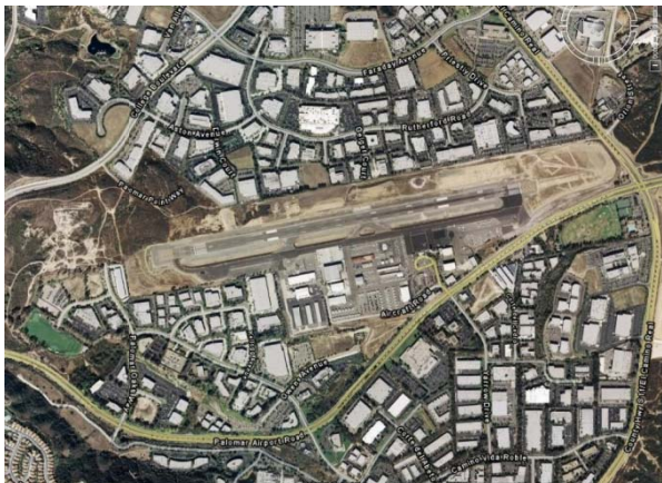
Aerial View of McClellan-Palomar Airport
