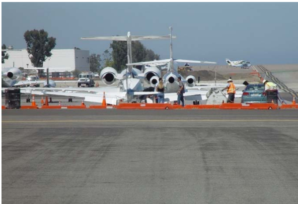
GA Apron Construction Activity (CRQ)
