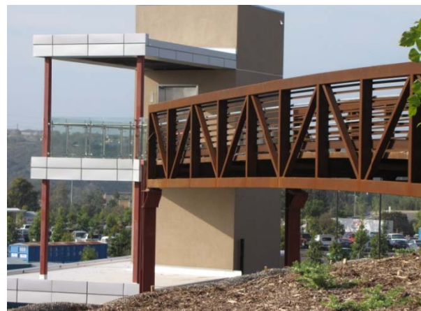
Lower Level Parking Pedestrian Bridge (CRQ)
