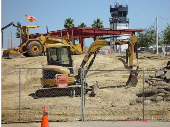
New Terminal Construction (CRQ)
