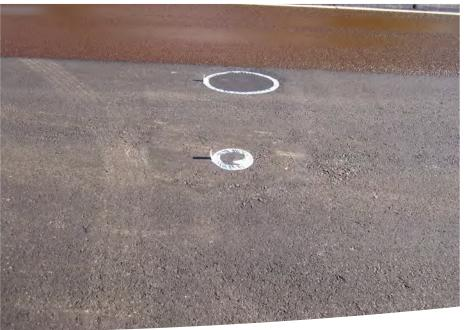
Protect and Mark all Utility Covers prior to Slurry Seal and/or Micro Surfacing.
