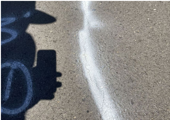
Photo 3-1-5: Close Up of Crack #1 (18 M)
