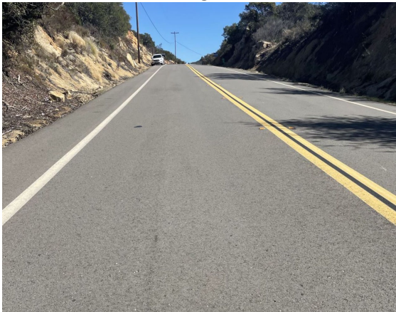
Photo 2-4-3: Skyline TT 18 Months. Overall, the road is in good condition
