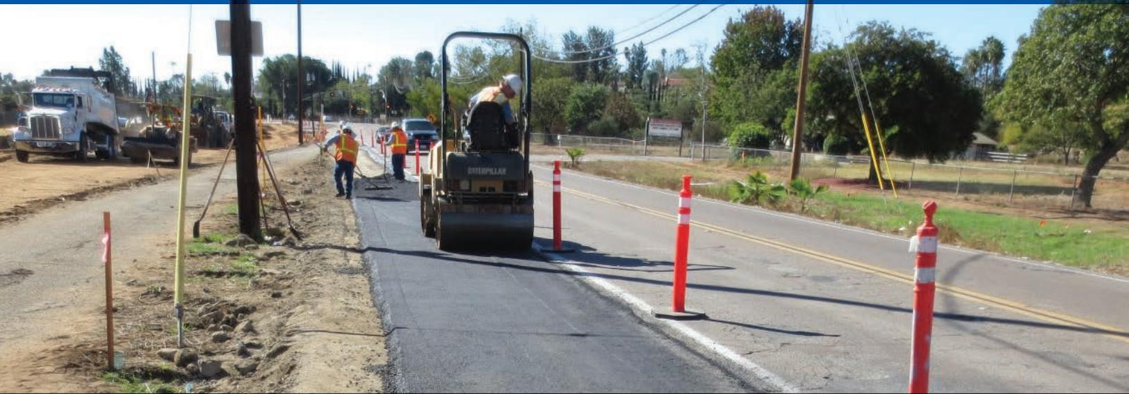
Crews place temporary asphalt concrete for pedestrians and bicyclists to use during construction.
