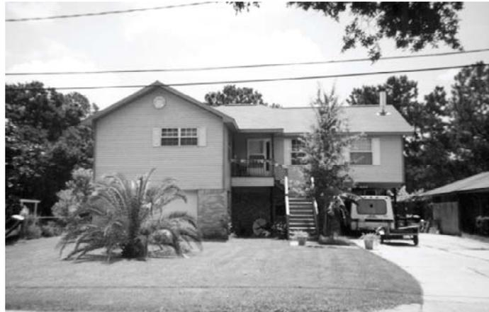
Retrofitted home elevated on extended continuous foundation walls.
