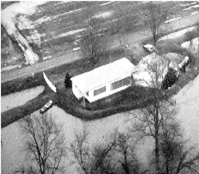
A home protected by a levee, which holds back the floodwaters shown in the lower half of the photograph. Note that the levee ties into high ground created by the road embankment.
