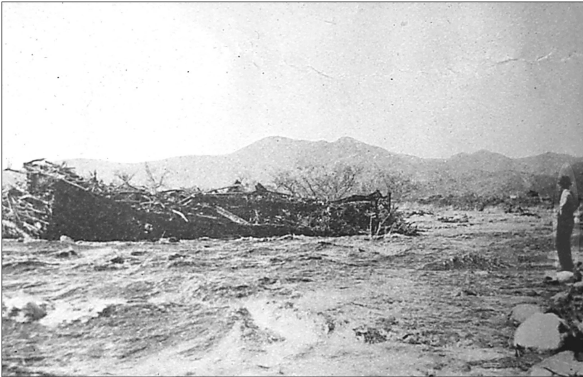
Wreck of Highway Bridge across San Luis Rey River at Pala after the Flood of January 1916
