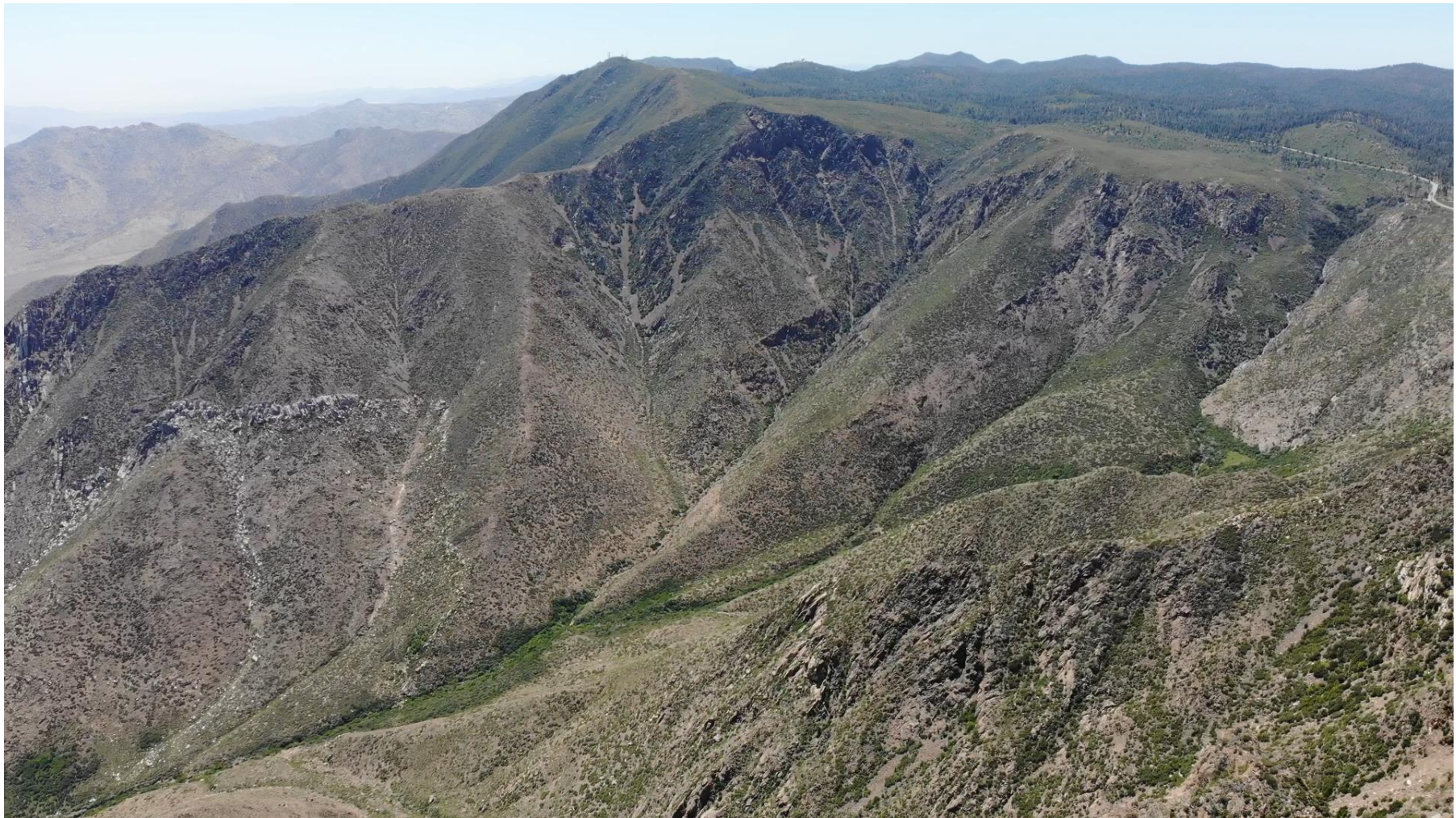
Figure 5-2. This June 2022 photo shows a small watershed in the Laguna Mountains with at least a 1% annual chance of debris flows, based on USGS data (Photo: J. Viducich, River Focus).
