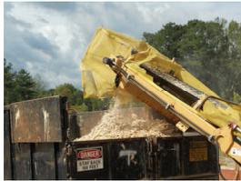
**Reuse materials on-site.** Grind materials such as wood, shingles, brick, and gypsum board that can be reused onsite. For example, ground wood waste provides a free source of mulch for landscaping, erosion and sediment control, delivery pads, and temporary paths or roads. Ground wood waste can also be used on landscape
