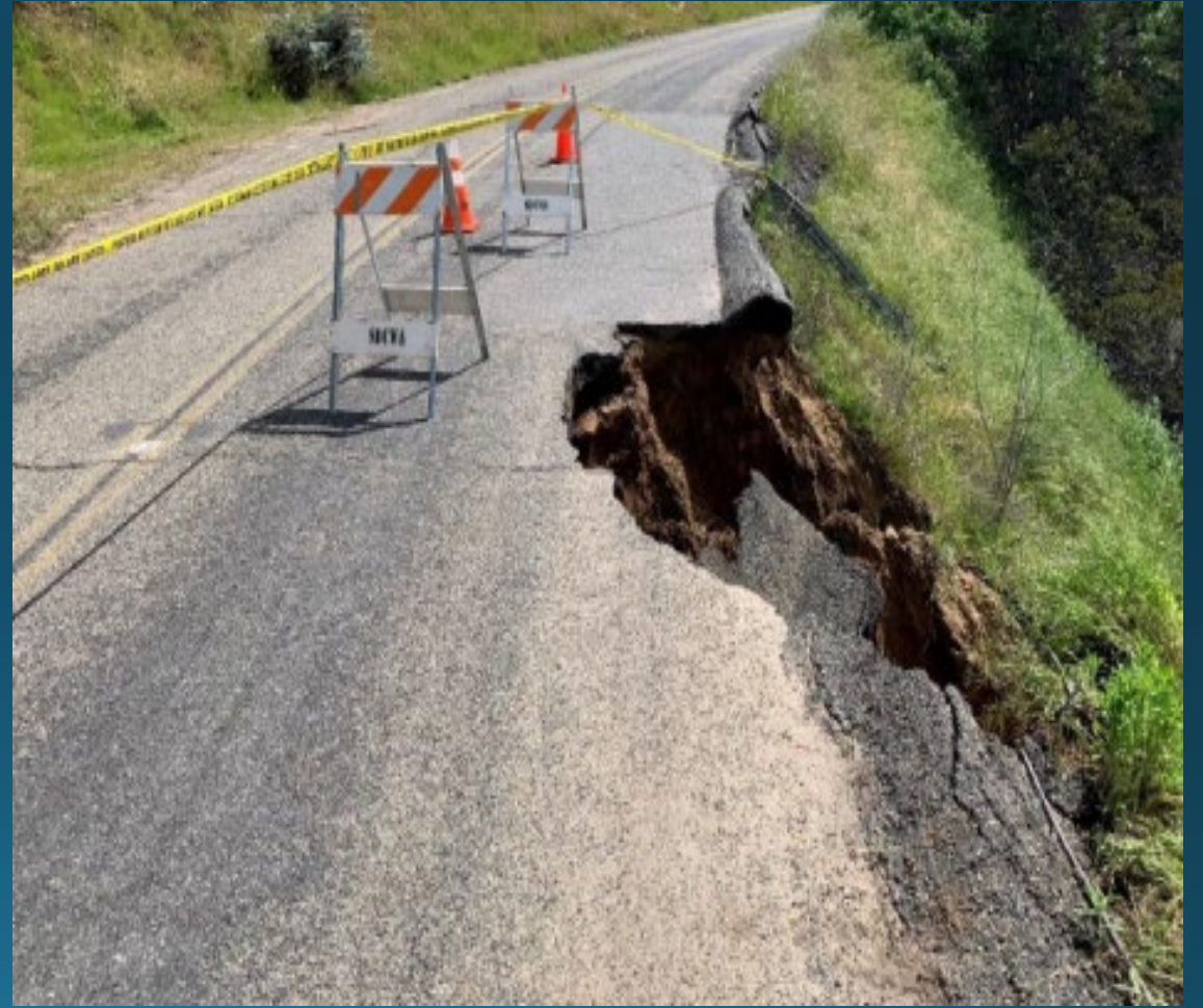
Sage Road failure, repaired summer 2023
