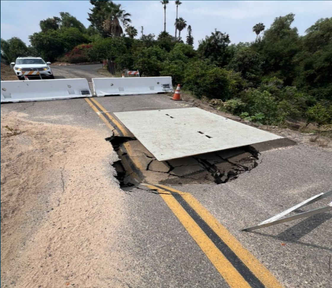
Sage road culvert failure, repaired Dec. 2024
