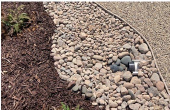
Buried overflow pipe that outlets to a rock dissipation area
