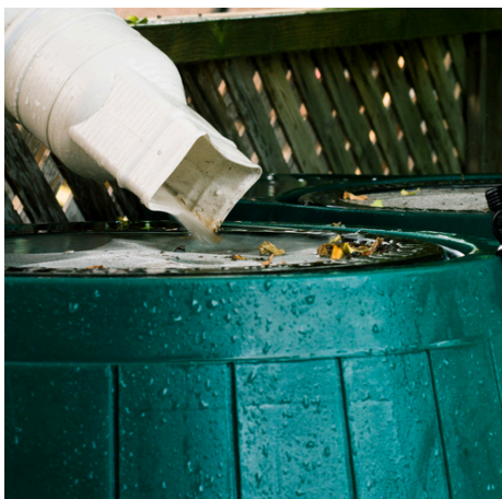
Debris and leaves on screening
