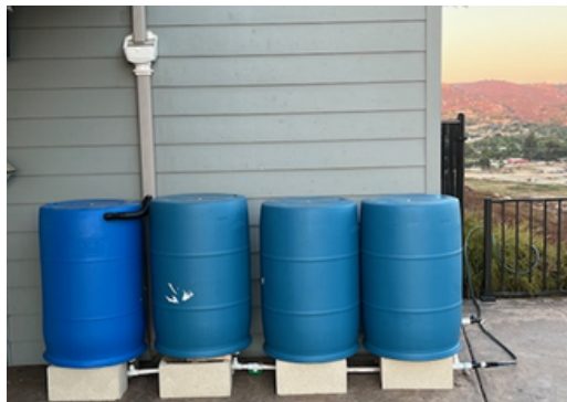
Four-barrel system with daisy chain configuration at the bottom
