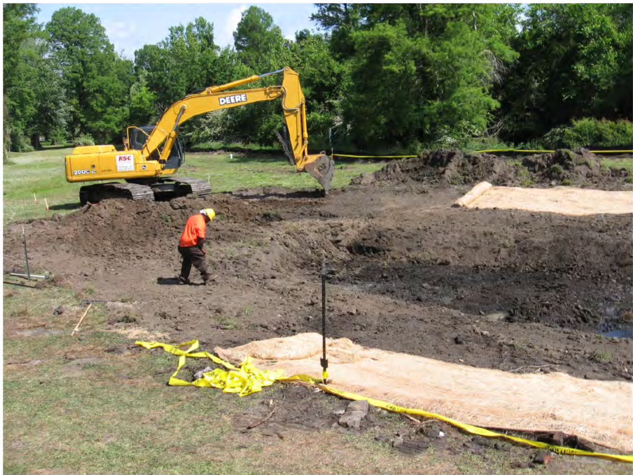
Figure 4-4. Heavy equipment (especially wheeled equipment) should be operated outside the excavated area to prevent compaction.
