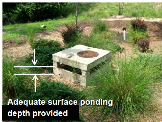
Figure 4-3. Accurate grading and outlet elevations must be provided to achieve intended hydrologic and water quality functions.
