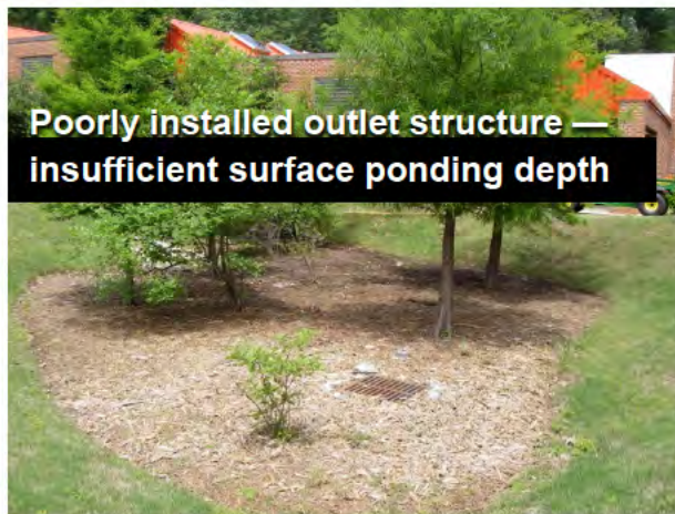
Figure 4-3. Accurate grading and outlet elevations must be provided to achieve intended hydrologic and water quality functions.
