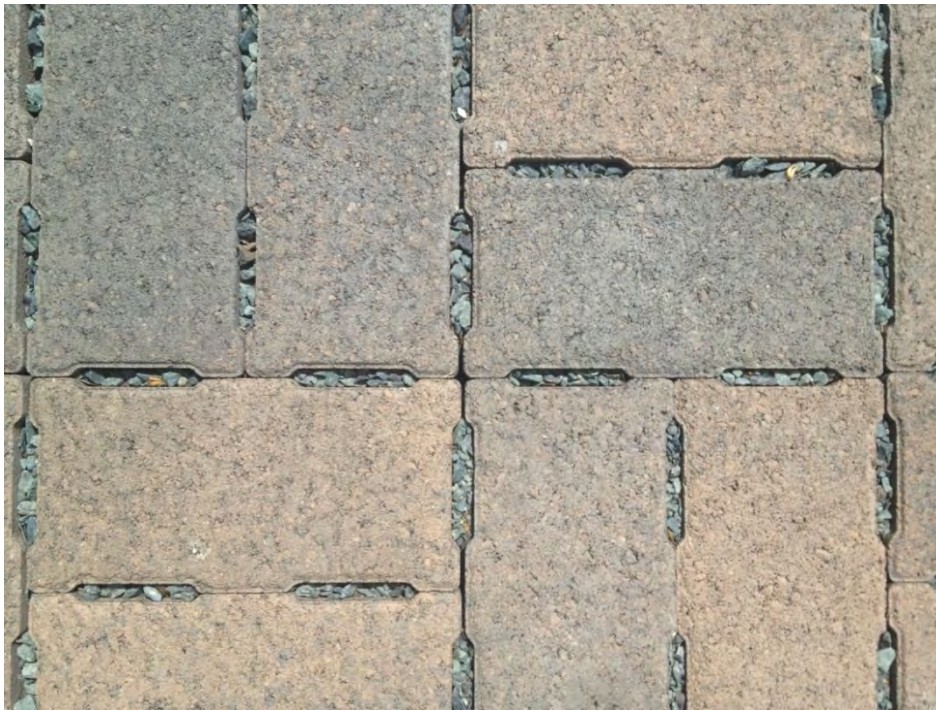
Figure 4-25. PICP was chosen as the surface course for this application. Bedding and joint fill material consists of washed ASTM No. 8.
