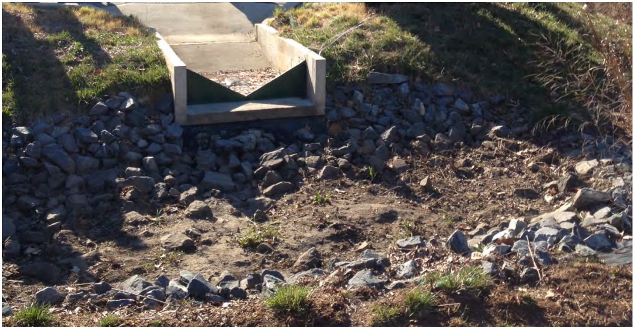
Figure 4-13. Inlet curb cut with a v-notch weir.
