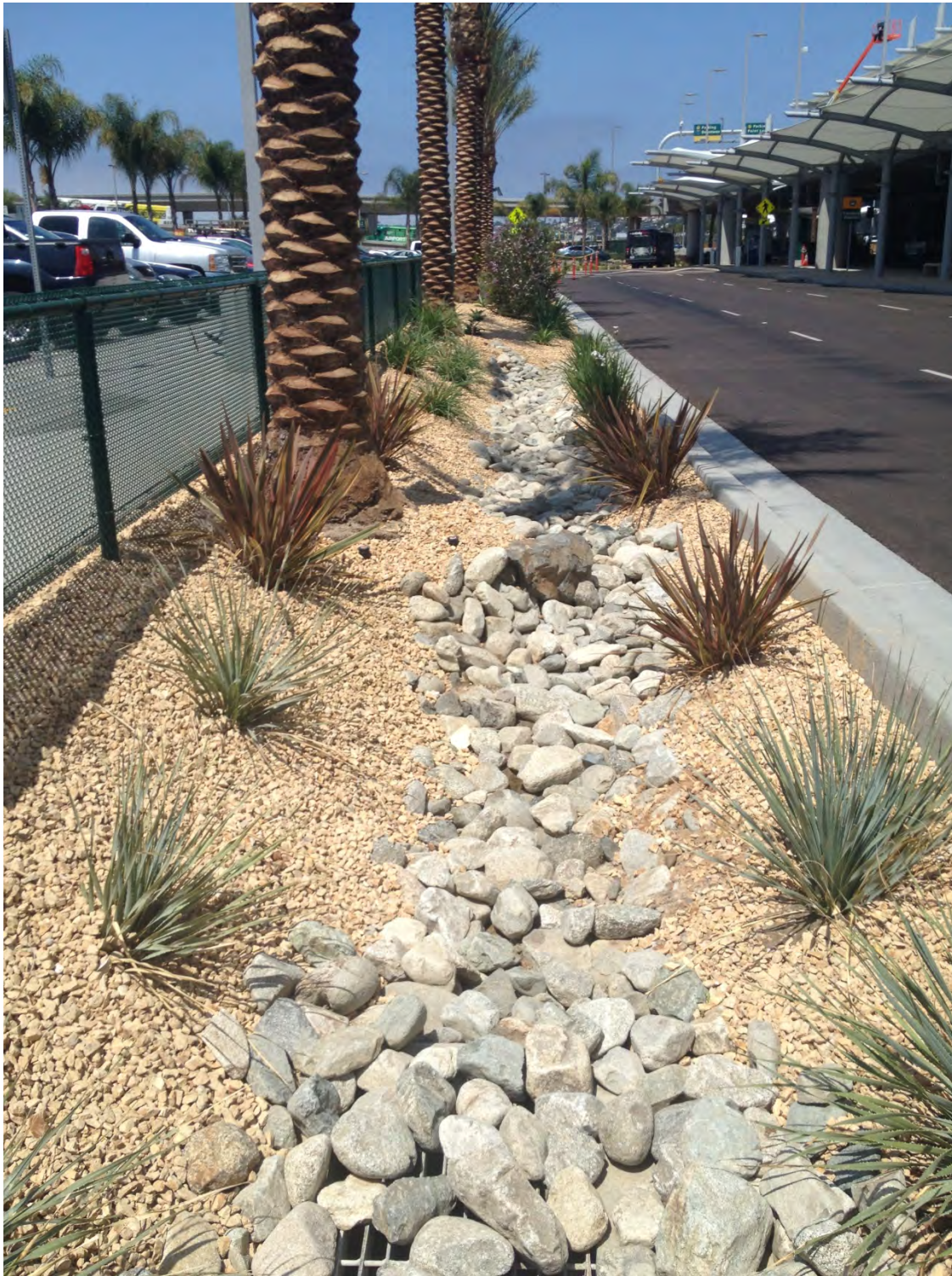
Figure 4-23. Cobble and gravel stabilize the surface of the rock infiltration swale and prevent scour of underlying soil media. The outlet structure in the foreground is elevated 2" above the bed of the rock infiltration swale to ensure that the design storm flow is retained and filtered through the media.
