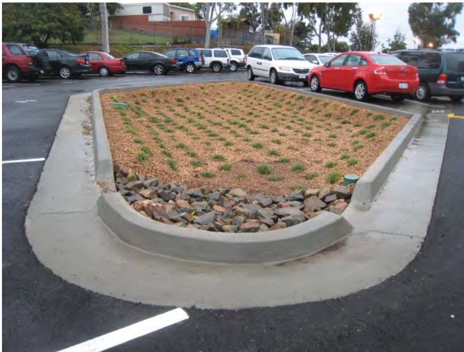
Figure 3-14. Bioretention parking lot island.
