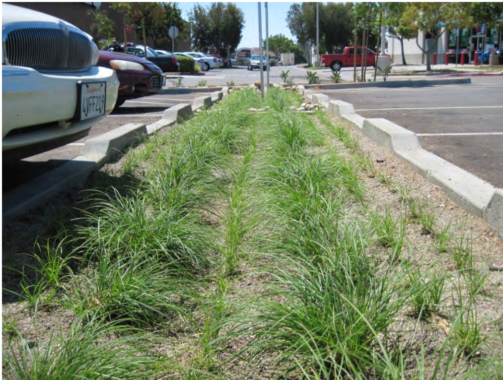
Figure 3-46. Vegetated swale.
