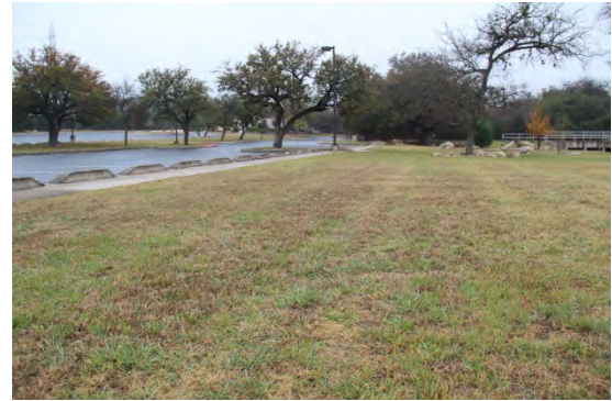
Figure 3-48. Vegetated filter strip.
