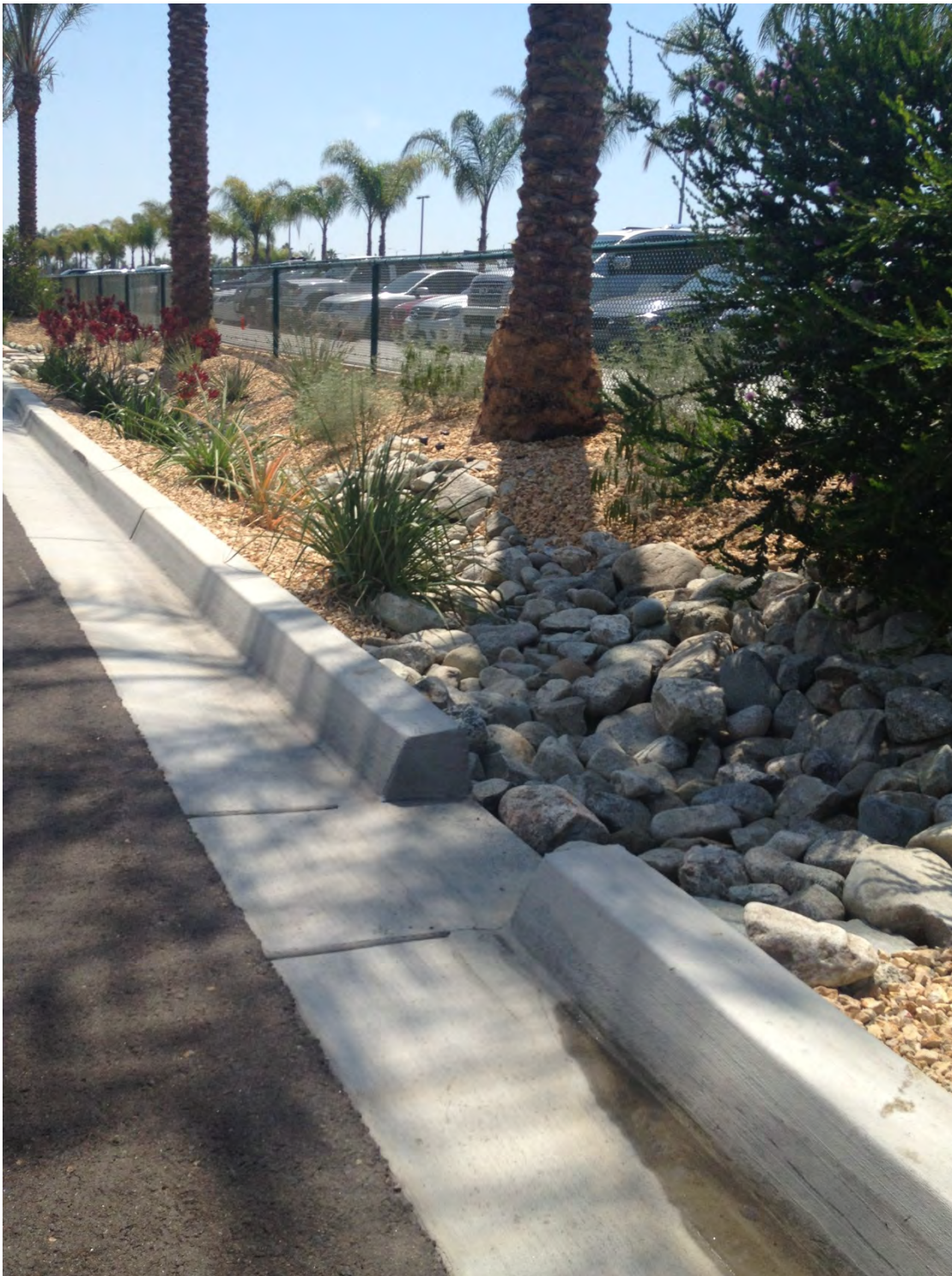
Figure 4-22. Curb cut and cobble energy dissipation at inlet to rock infiltration swale.
