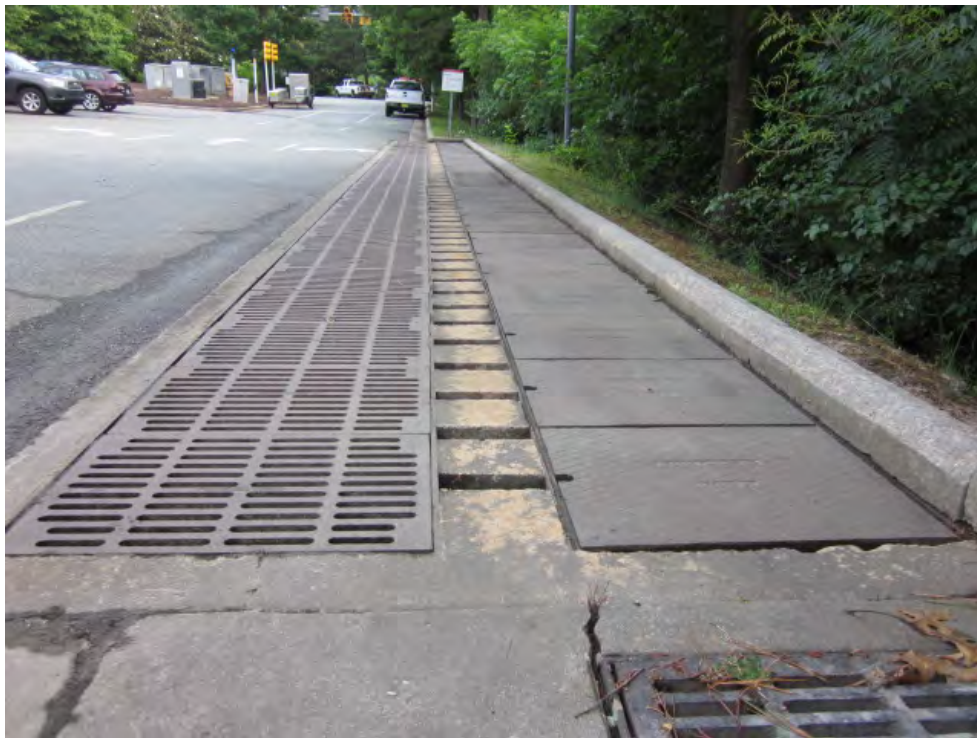
Figure 3-37. Subsurface sand filter in parking lot.
