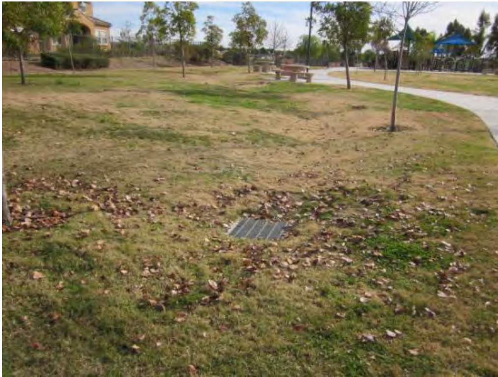
Figure 3-46. Vegetated swale.
