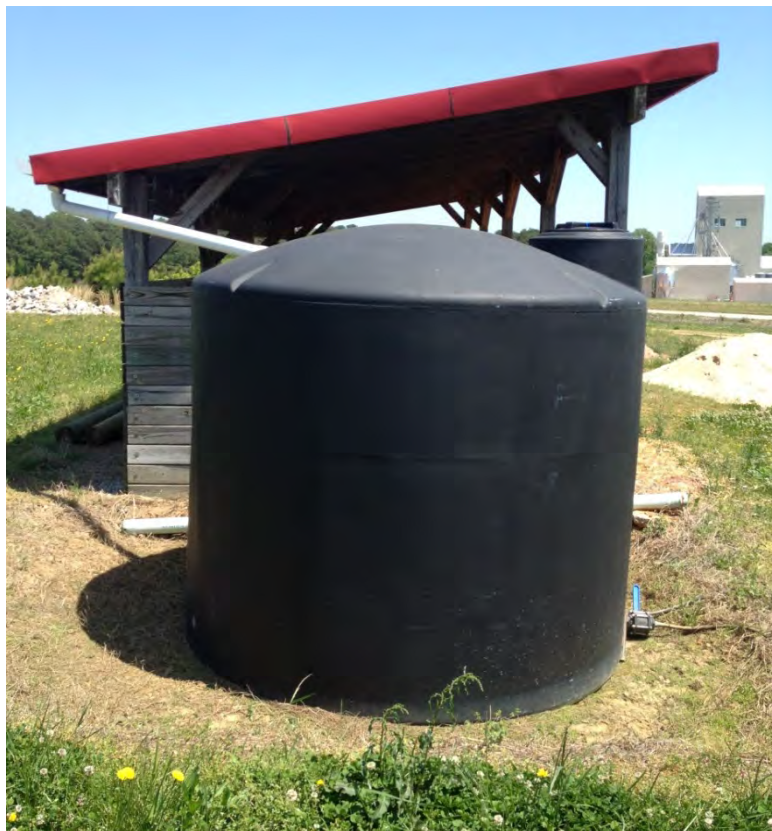
Figure 3-39. Typical plastic cistern.
