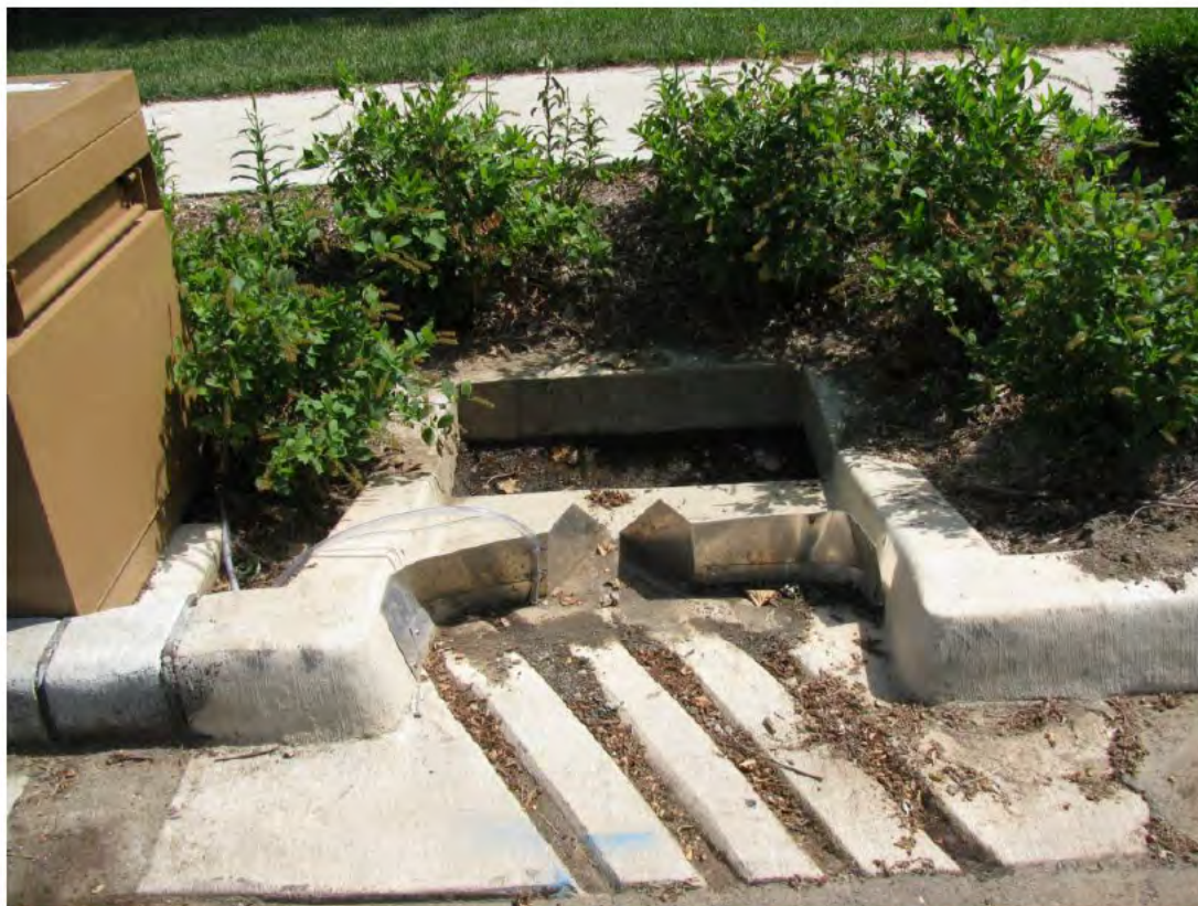
Figure 4-17. Poorly installed H-flume at the inlet to a bioretention area in which the invert of the weir is too low and tailwater from the bioretention will interfere with measurement.
