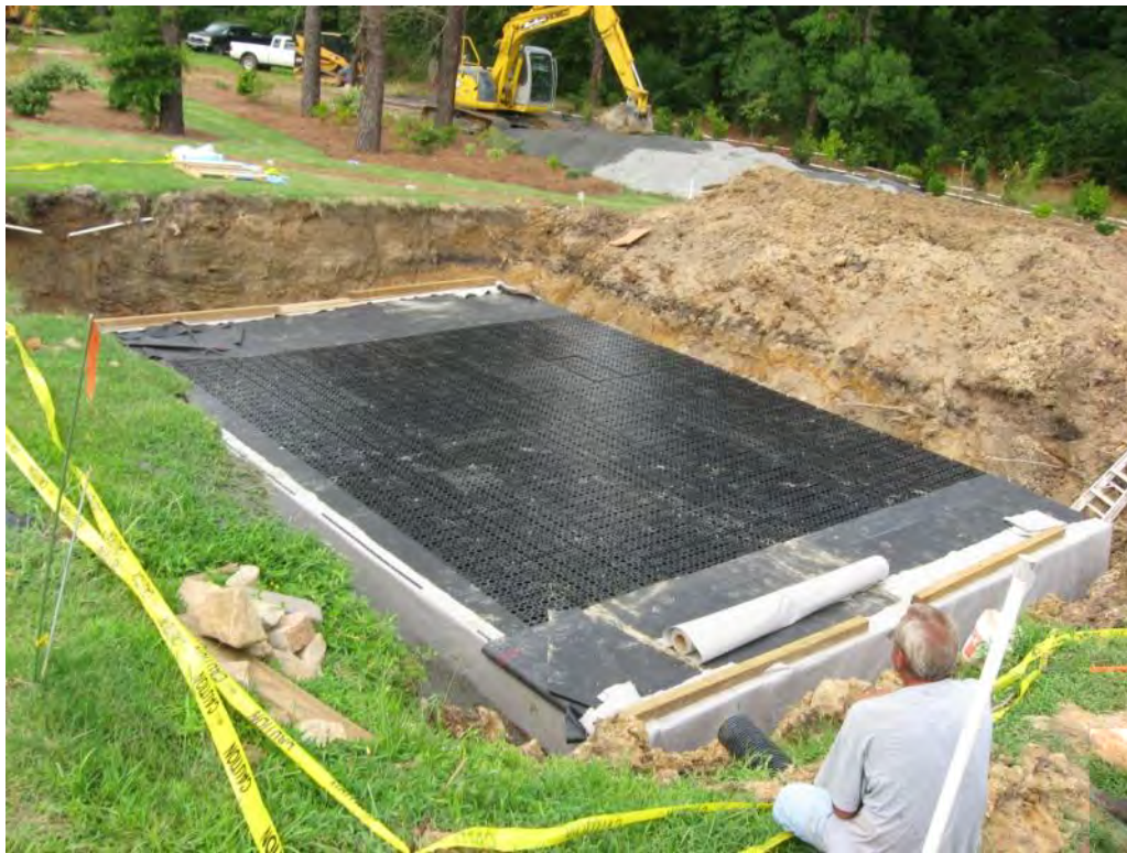
Figure 3-42. Below-ground cistern.
