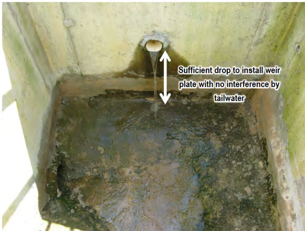
Figure 4-16. Example of a bioretention underdrain outlet with sufficient drop to install a flow monitoring weir without encountering tailwater.
