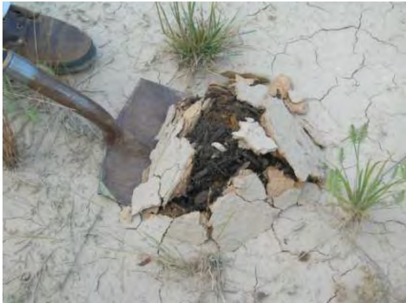
Figure 4-6. Bioretention area clogged with sediment.
