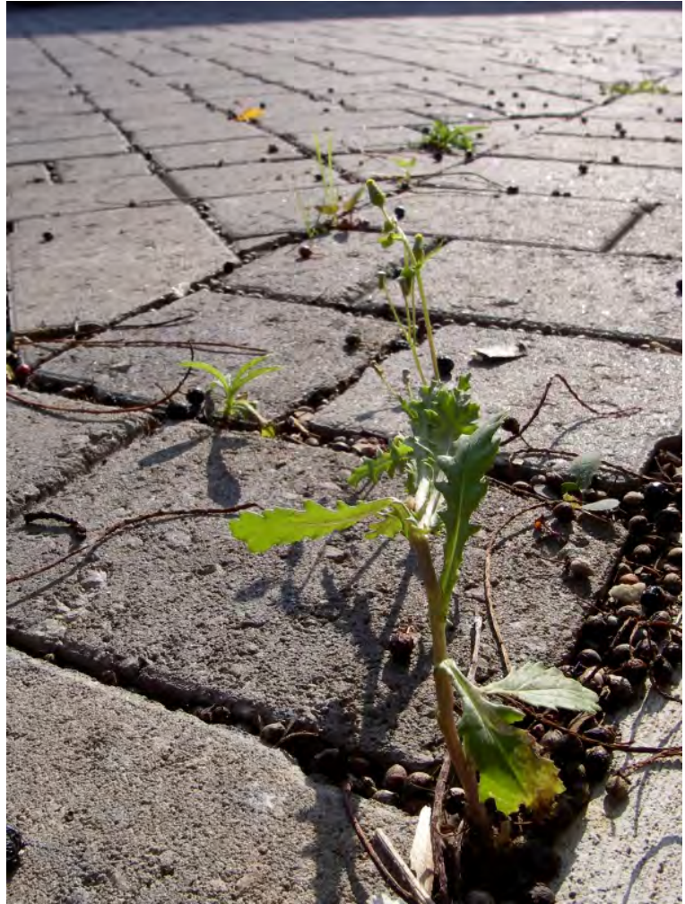
Figure 4-9. Plant growth, debris buildup, and puddles indicate that permeable pavement is clogging. Prompt maintenance should be performed to prevent joints from fully sealing.
