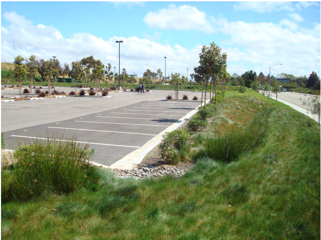
Figure 2-8. Parking lot that drains to a vegetated swale.
