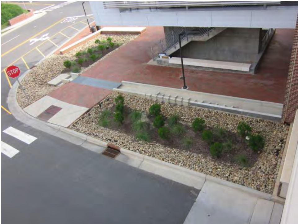
Figure 3-16. Parallel bioretention areas treat parking structure runoff conveyed by a concrete flume.
