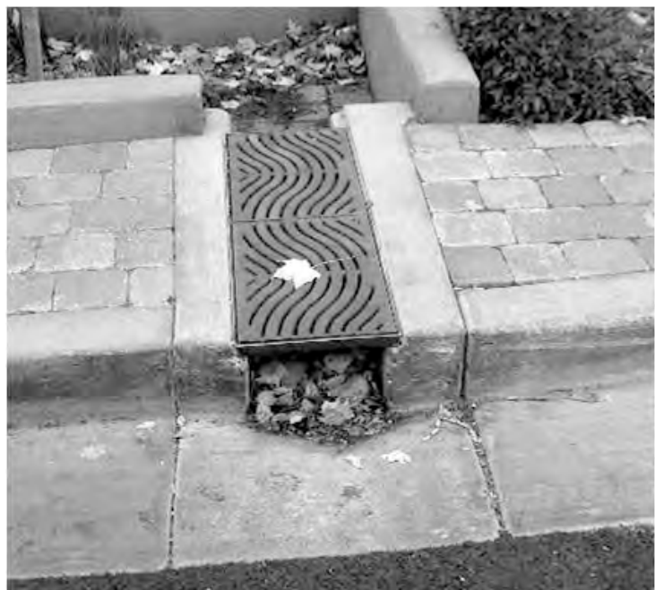
Figure 4-7. Inlet sump to remove gross solids.
