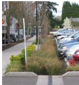
Bioswale adjacent to parking and sidewalk
