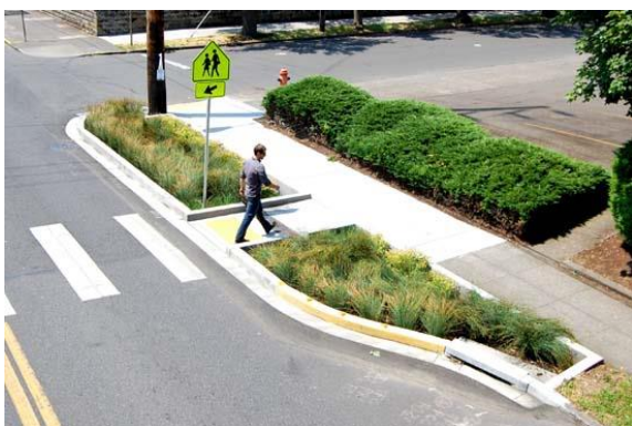
Bulb-out planter box at intersection
