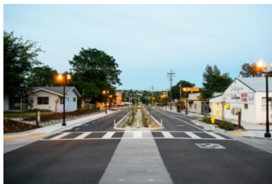
Roadway with depressed median and bulb out planter at intersection
