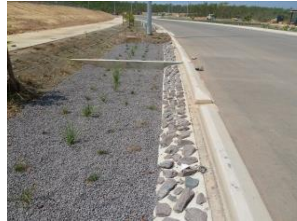
Rock swale adjacent to road
