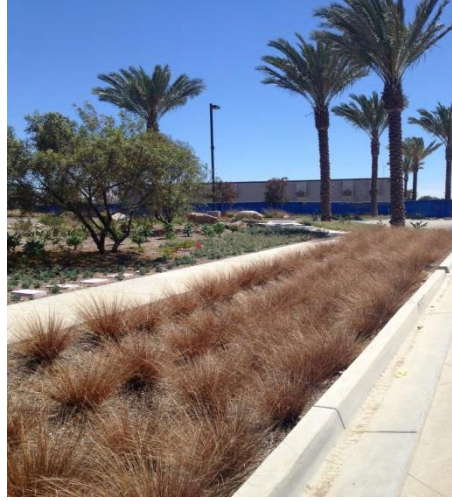
Swale adjacent to road
