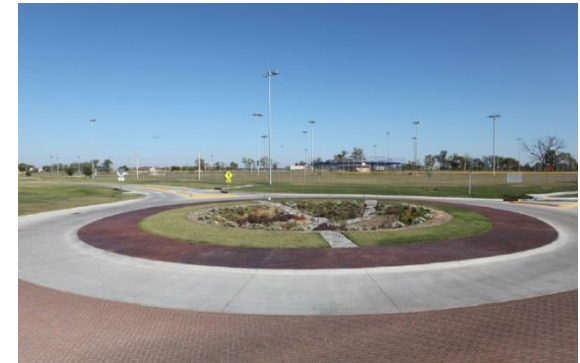
Street view of same roundabout
