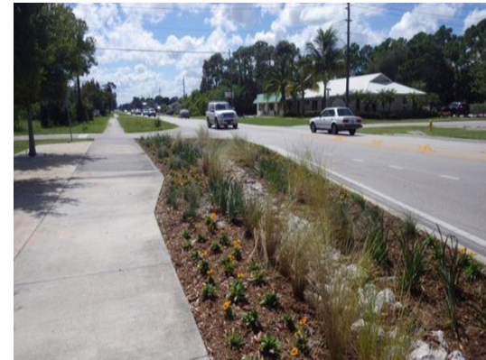
Swale adjacent to road
