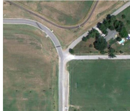
Aerial view of rural intersection before roundabout
