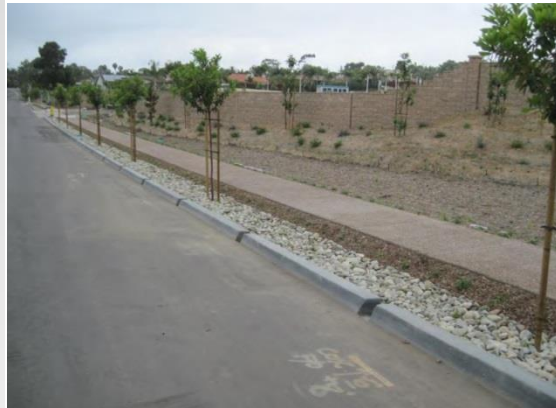
Rock swale adjacent to road
