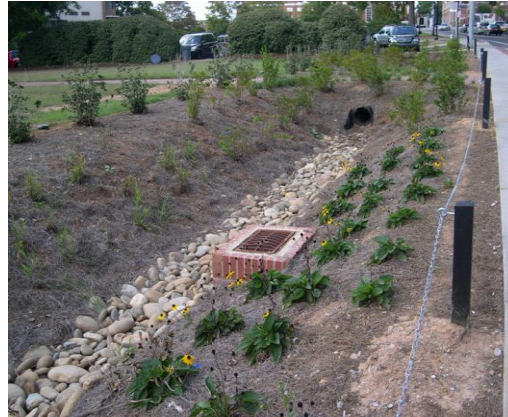
Swale outside of parking lot
