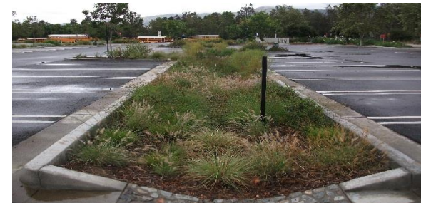
Swale in Island
