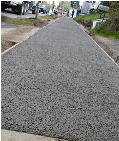
Pervious concrete sidewalk
