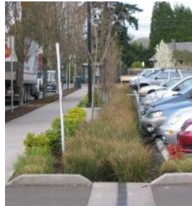
Bioswale adjacent to parking and sidewalk
