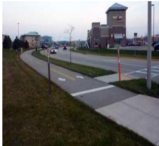
Porous asphalt pathway
