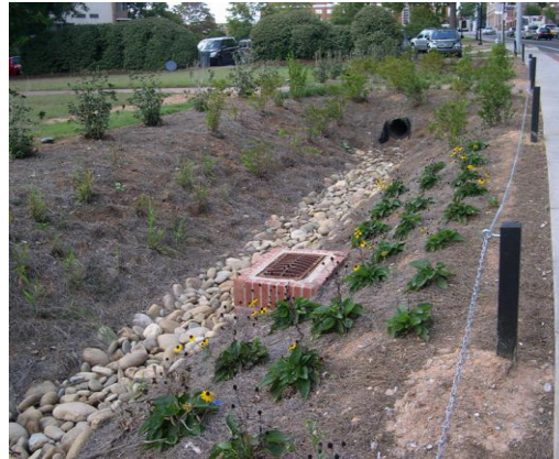
Swale outside of sidewalk and road
