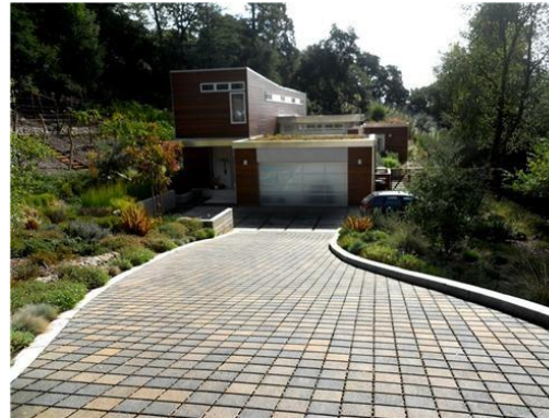
Permeable pavement driveway
