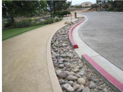
DG pathway with rock swale
