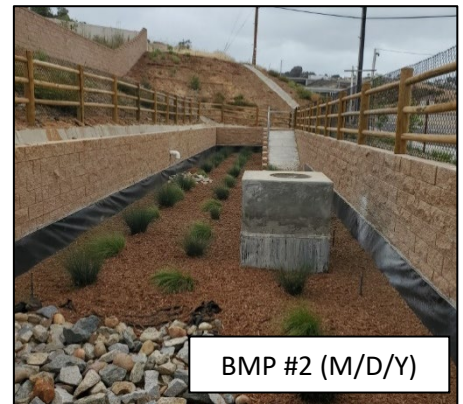
Finished BMP with soil media, surface mulch, and vegetation
