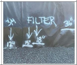
12" of ¾ washed aggregate (Pic of each layer after filling to pre-measured lines)
