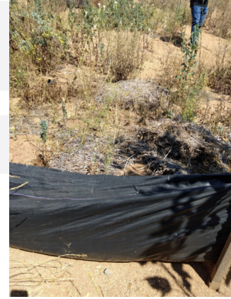
Silt fence not installed correctly
