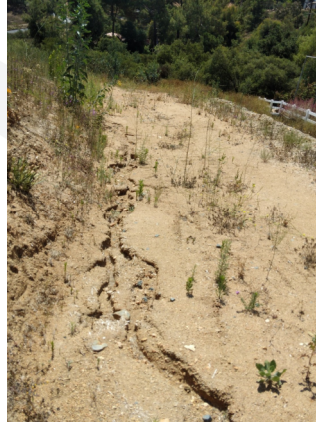
Long Term Erosion without BMPs
