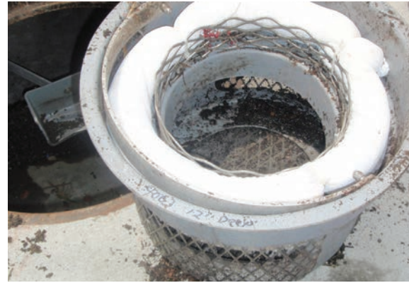
Drain Insert BMP
