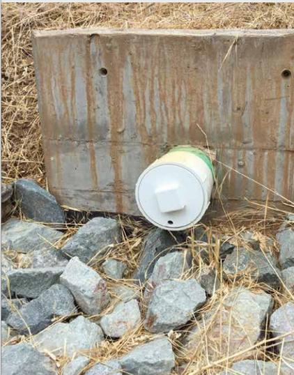
*Underdrain Cap with Orifice*
