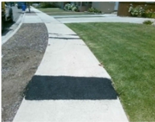
Figure 3. Ramped Sidewalk
