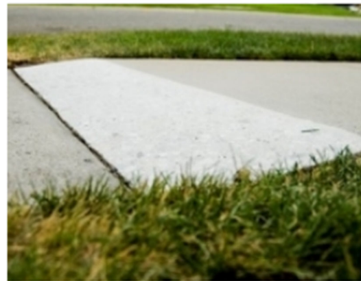
Figure 4. Sliced Sidewalk
