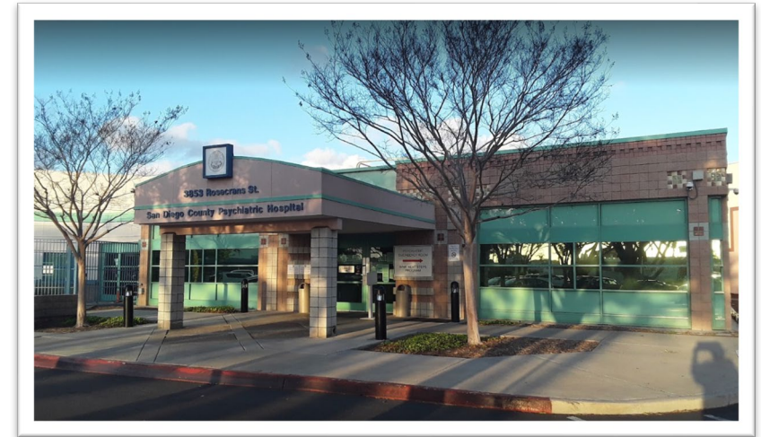
Picture of the San Diego County Psychiatric Hospital (SDCPH).
