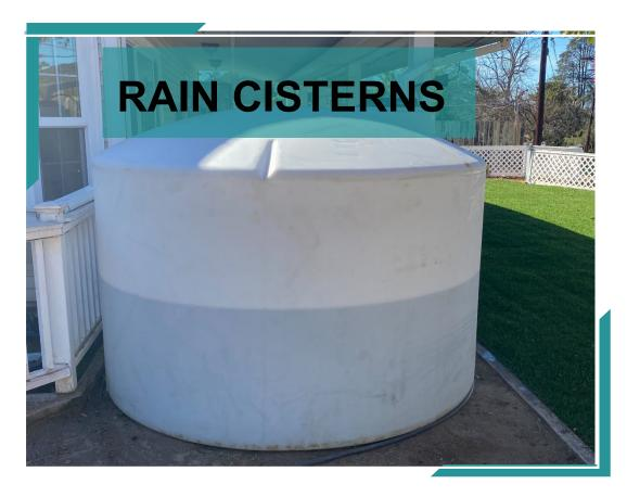
Rain cisterns are large rain barrels that can capture a lot more rainwater. Cisterns can hold between 200 and 5,000 gallons.
