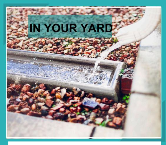
You can redirect a downspout to send water directly into a lawn or landscaped area. The area should be half the size of the area it is capturing water from.
