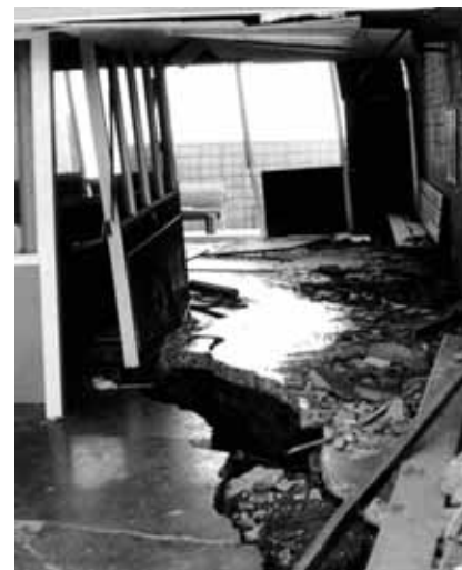
LA County Juvenile Hall, Sylmar, California damaged by liquefaction during the magnitude 6.6 San Fernando earthquake of February 9, 1971. The broken floor is due to settling of the earth and is not the fault itself. Photo by Jack Meehan, structural engineer.
