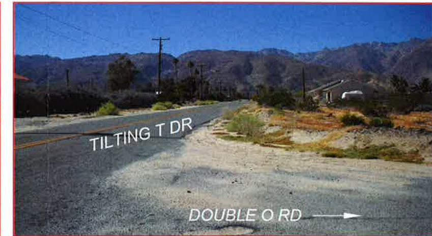
② SIGHT DISTANCE LOOKING AT WESTERLY DIRECTION = 500'+
