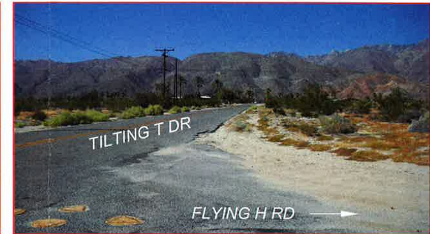
② SIGHT DISTANCE LOOKING AT WESTERLY DIRECTION = 500'+
