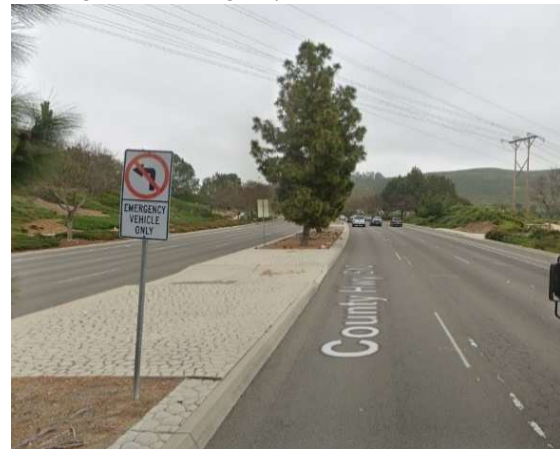
Image 8: Conceptual design of raised median with mountable stamped concrete
