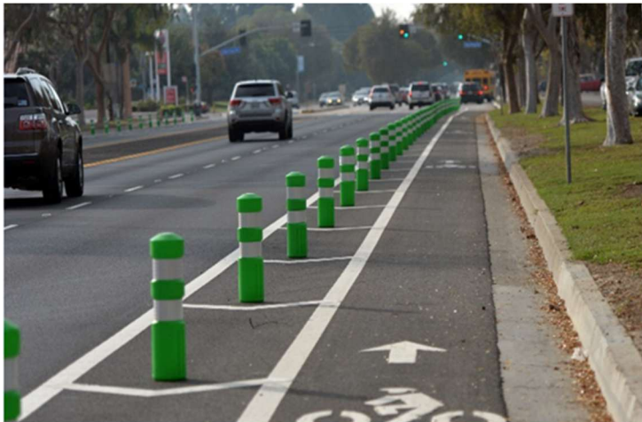
Photo 29: Example of a Class IV bikeway
