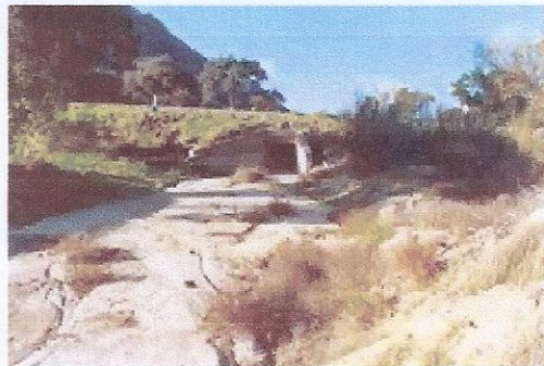
Box culvert at highway crossing.
