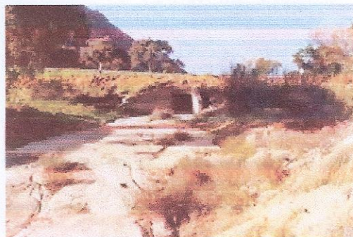
Box culvert at highway crossing.
