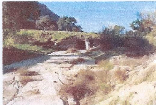
Box culvert at highway crossing.
