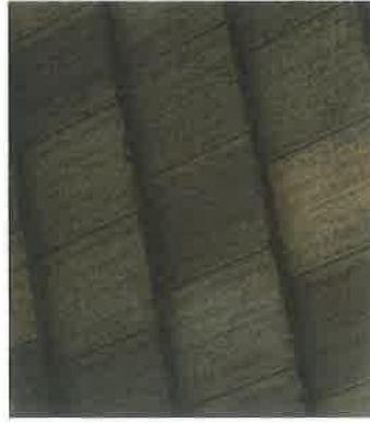
ROOF FLAT TILE
