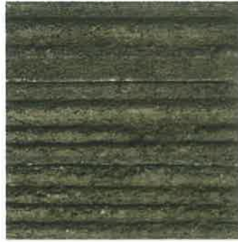
ROOF FLAT TILE
