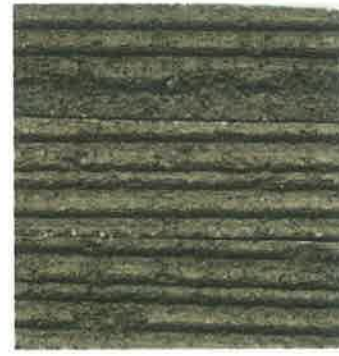
ROOF FLAT TILE
