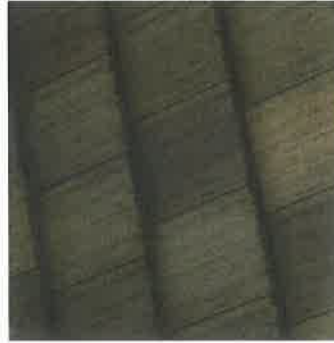
ROOF FLAT TILE
