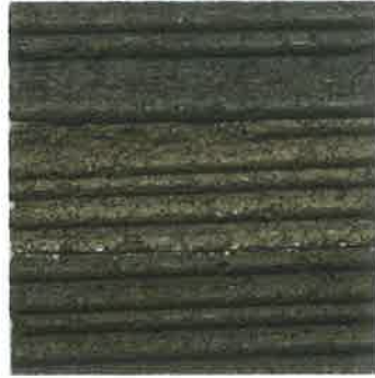
ROOF FLAT TILE
