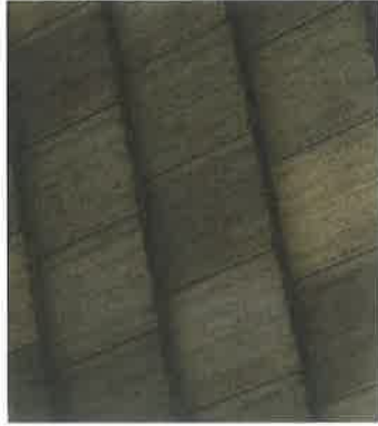
ROOF FLAT TILE
