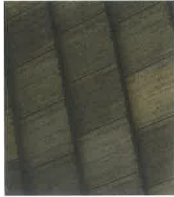
ROOF FLAT TILE
