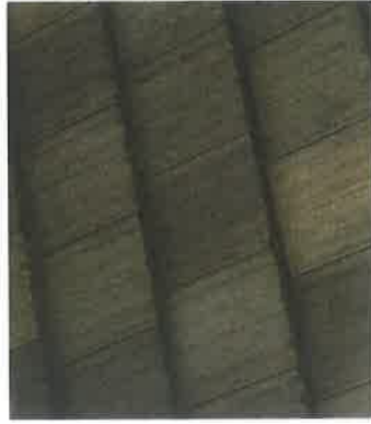
ROOF FLAT TILE
