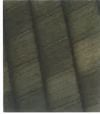
ROOF FLAT TILE
