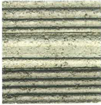
ROOF FLAT TILE
