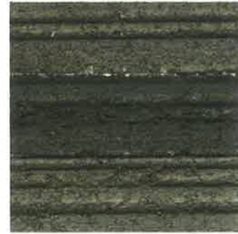
ROOF FLAT TILE
