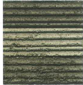
ROOF FLAT TILE
