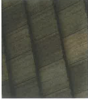
ROOF FLAT TILE
