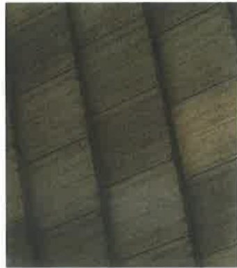
ROOF FLAT TILE
