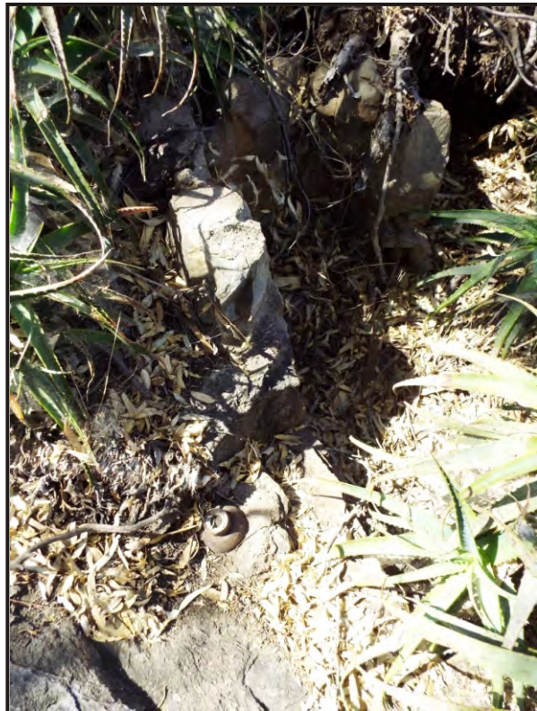
b. Chimney-like Structure and Metal Attachment, Looking North (PR-05861-058)
