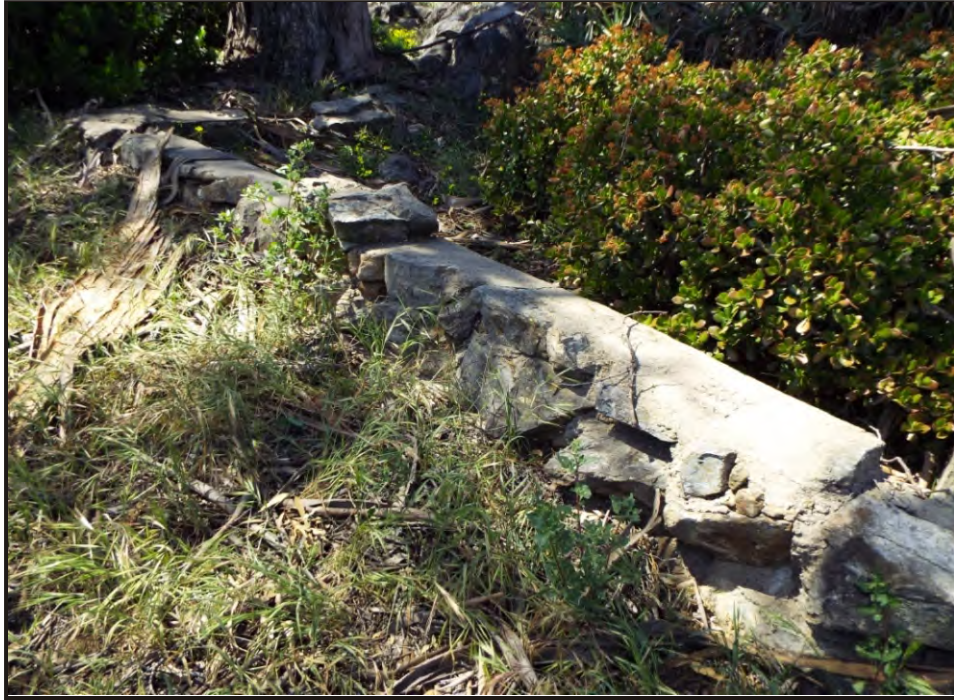
a. P-35-035639 Wall Structure Overview, Looking Southwest (PR-05355-015)
