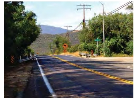
Existing road without pedestrian or bicycle facilities.
