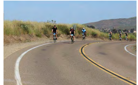
Roadway with one lane per direction and no median
