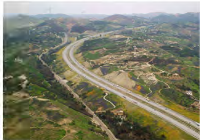
Interstate 15 looking north
