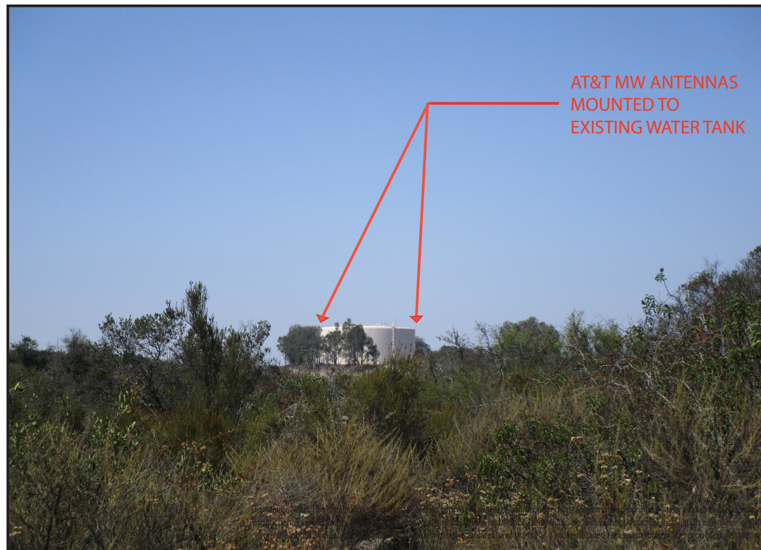
SITE AFTER INSTALLATION
