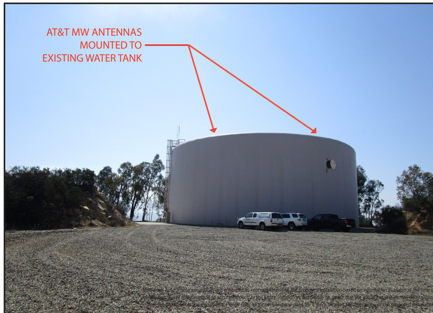
SITE AFTER INSTALLATION
