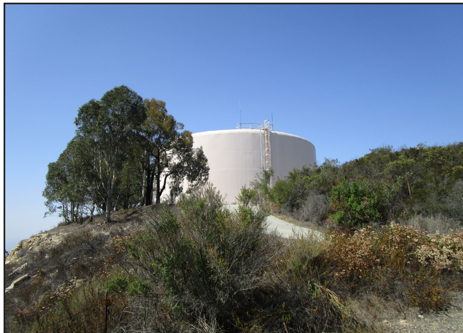
SITE PRIOR TO INSTALLATION
