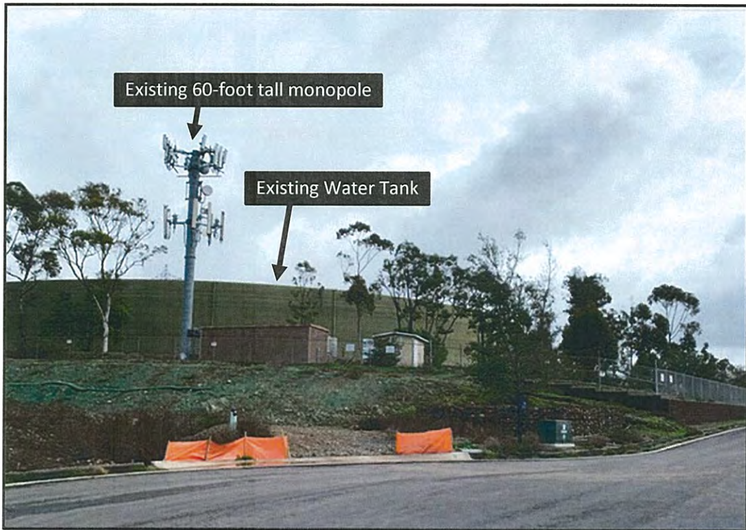
Figure 1: Existing 60-foot tall monopole looking toward project site.
