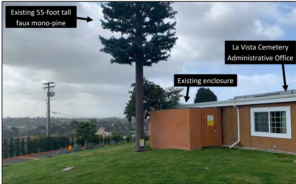
Figure 3: Existing 55-foot tall faux mono-pine and enclosure.
