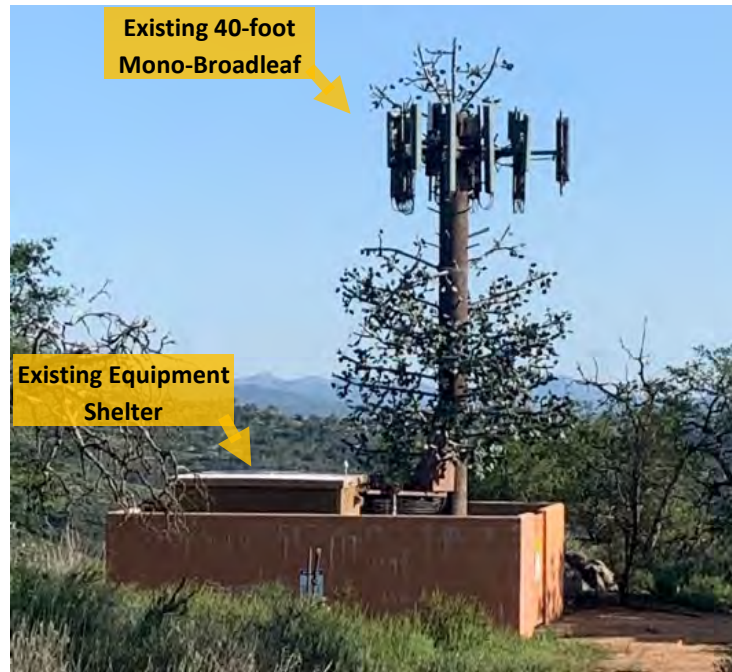
Figure 1: View of the existing mono-broadleaf tree and equipment enclosure, looking west.
