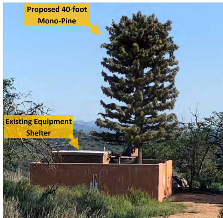
Figure 2: View of proposed 40-foot-tall mono-pine and equipment enclosure, looking west.
