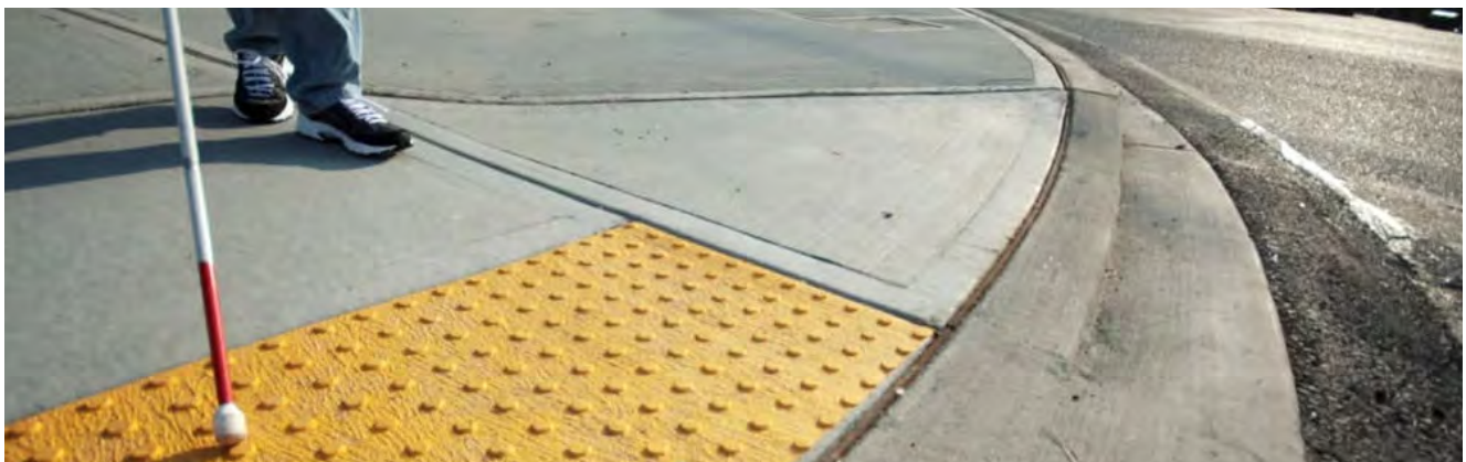
Example curb ramp and truncated domes
