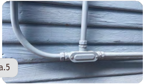
Surface mounted utility conduit
