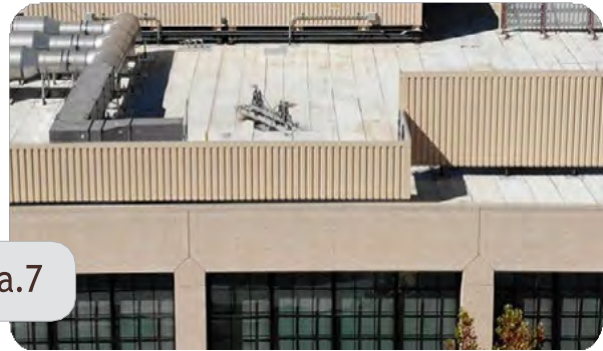
Screened Rooftop Mechanical Equipment
