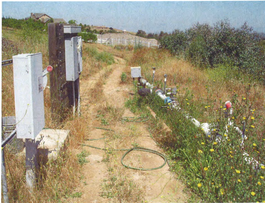
Photograph #5 Private well located on northeast property boundary.
