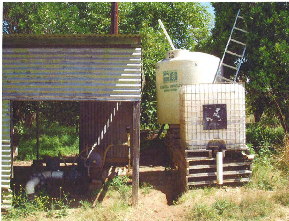
Photograph #1 Aboveground storage tank (AST) containing fish emulsion located at 32542 Aquaduct Road in middle of Site.
