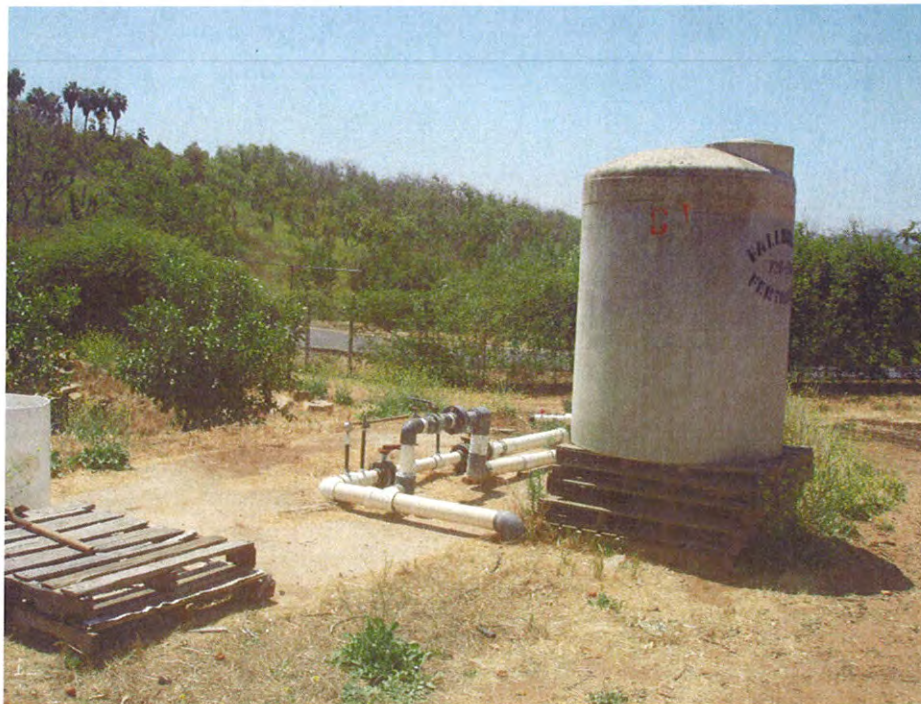
Photograph #4 AST located on 31817 Via Ararat Drive, near outfall at south boundary.
