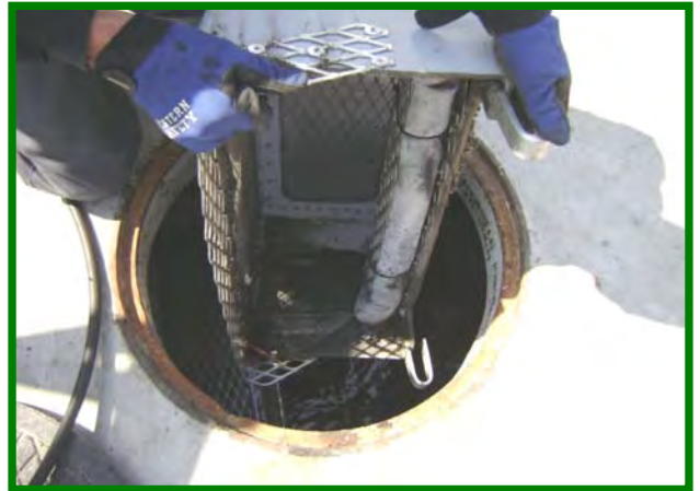
Remove Catch Basin Filter
