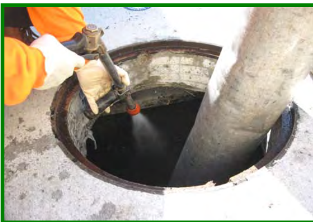
Vacuum out the Sediment Chamber
