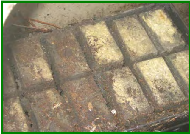
Remove Spent BioMediaGREEN Filter Blocks
