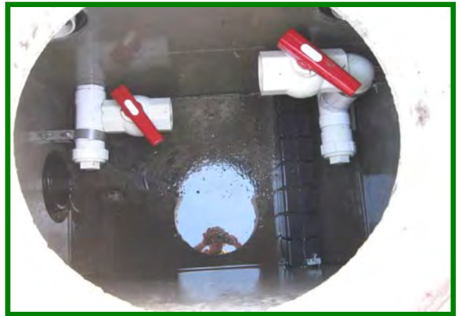
Open Discharge Chamber Lid to Assess Wetland Media Flow Rate and Replace Drain Down Filter Near Bottom
