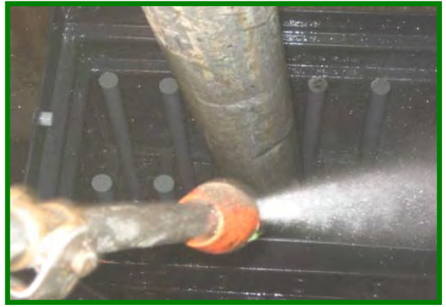
Spray Down and Clean Cartridge Filter Housing
