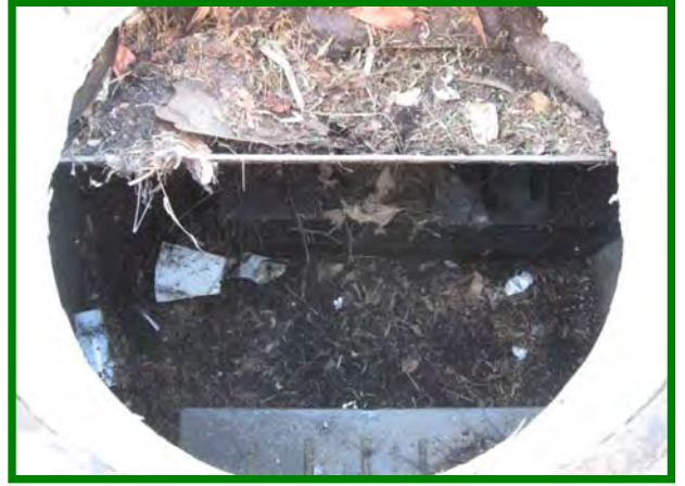
Assess Pollutant Loading in Catch Basin Filter and Sediment Chamber
